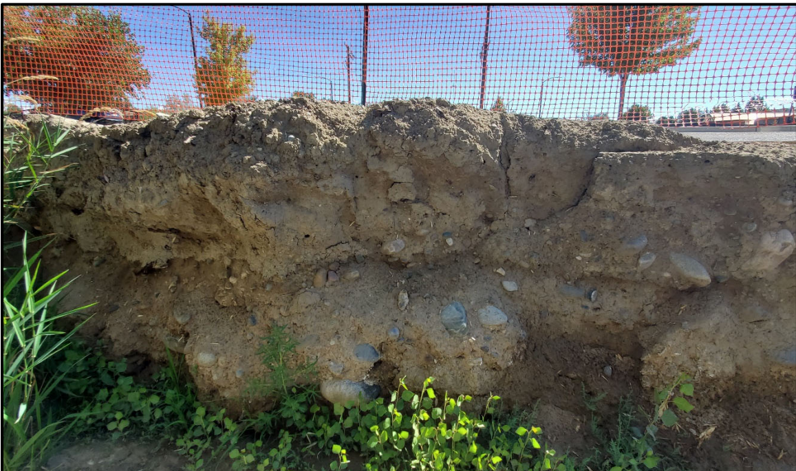
Fill Behind Gabion Wall near Boring B-3 View Towards the East
