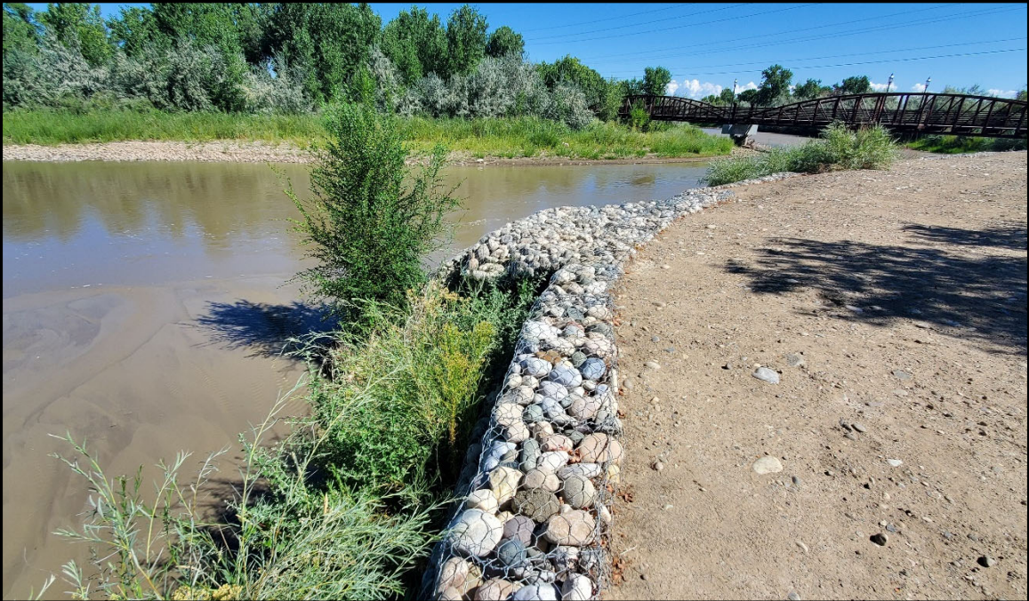
Gabion Wall near Boring B-4 View Towards the Northeast
