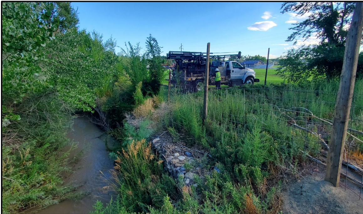
Drill Rig at Boring B-1 View Towards the North
