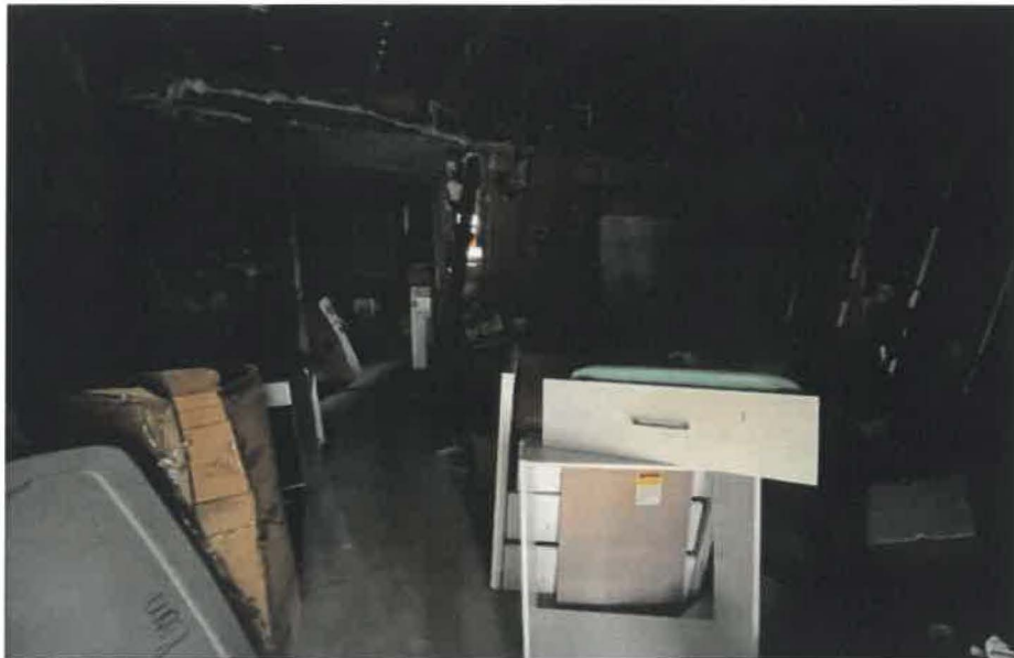
Inside of structure
