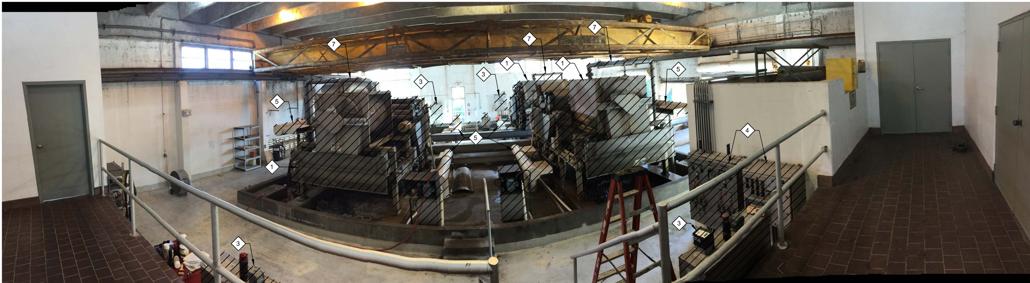
2 PHOTO SHOWING BFP No. 1, BFP No. 2, ODOR CONTROL DUCTWORK, SULDGE FEED PIPING, WASHWATER PIPING ON WEST SIDE OF DEWATERING SYSTEM MD01
