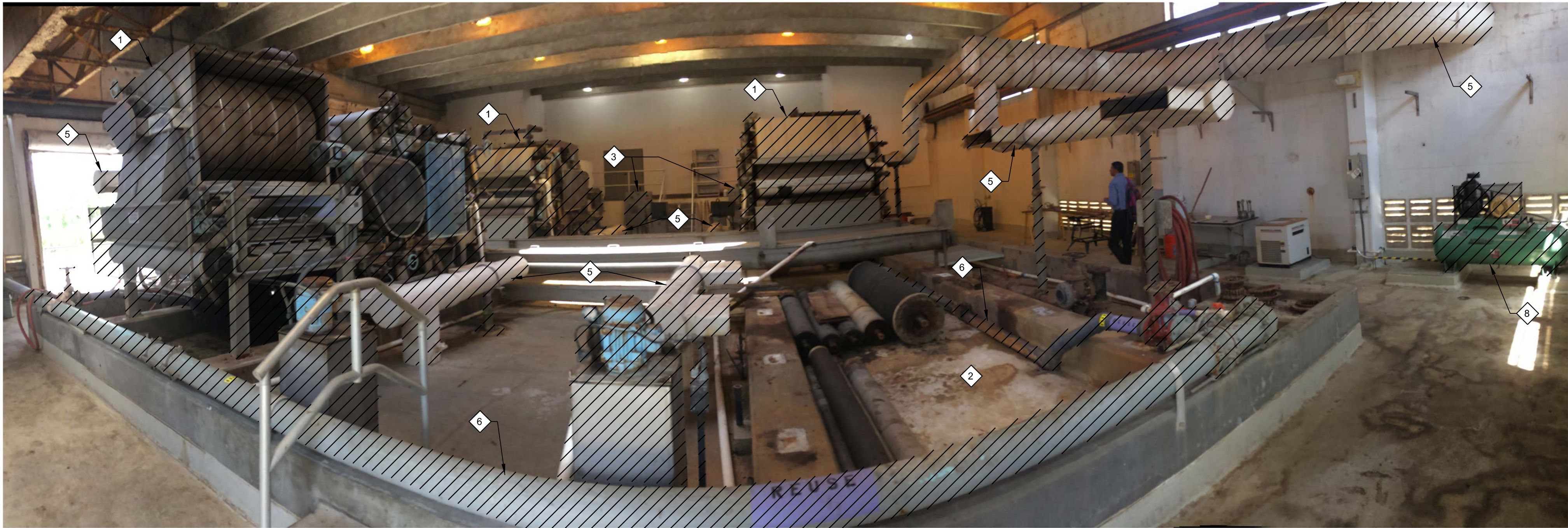
1 PHOTO SHOWING BFP No. 4, ODOR CONTROL DUCTWORK, SULDGE FEED PIPING, WASHWATER PIPING ON EAST SIDE OF DEWATERING SYSTEM MD01
