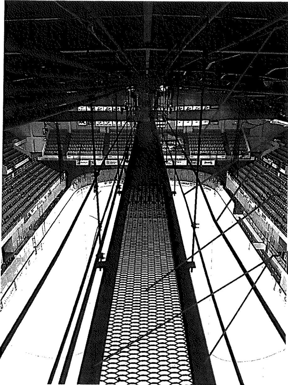
Hangers and vertical rails for guardrails
