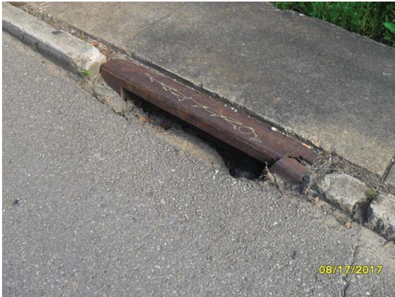
Catch basin to be replaced
