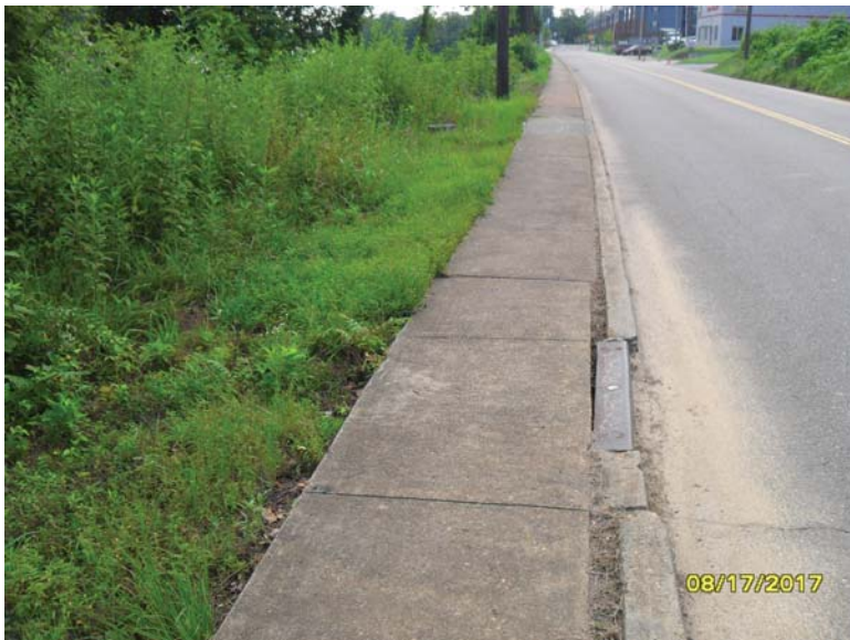
Catch basins to be removed
