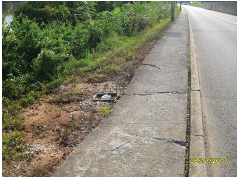
Sanitary clean out to be adjusted
