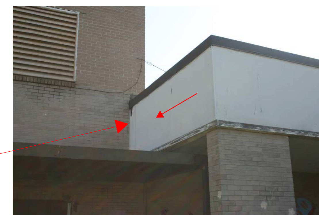
SIDING ENDING POINT
