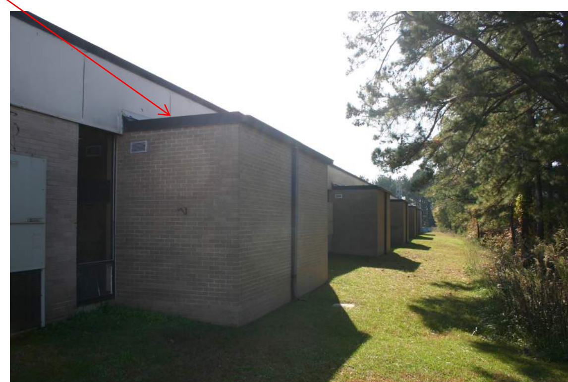
WEST ELEVATION (LOOKING SOUTH)
