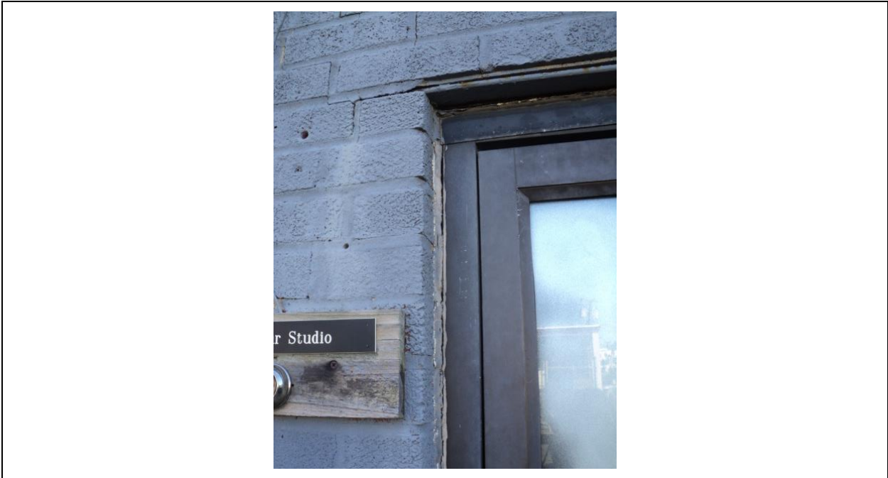
Homogeneous Material No. 13 – Non-ACM Grey Exterior Door caulk located outside the Inner Ear Studio
