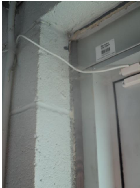
Homogeneous Material No. 2 – Non-ACM Grey Caulk located at the Interior Door in the 2 nd Floor Front Mezzanine Area
