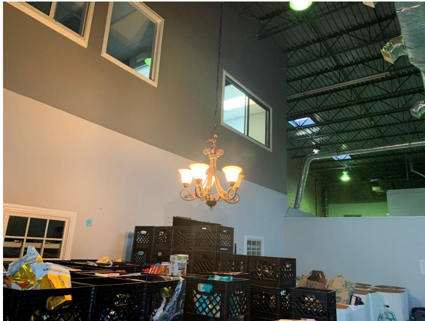
Typical fluorescent Bulb Lighting at the Subject Property
