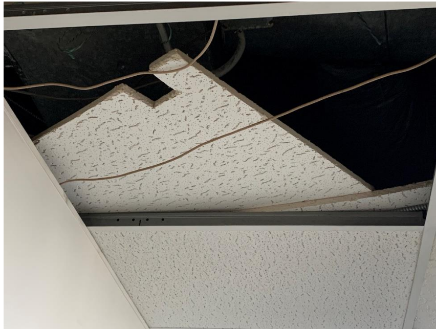
Homogeneous Material No. 3 – Non-ACM 2’X4’ White Textured Lay-in Ceiling Tile (dots with dashes design), located in all of 1 st floor and 2 nd floor front Mezzanine Plus part of back Mezzanine Area
