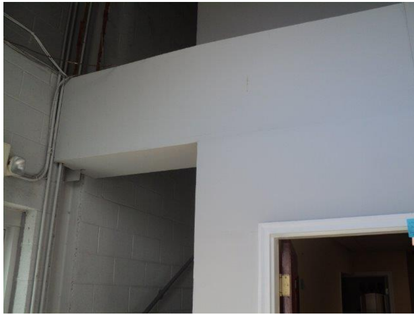
Homogeneous Material No. 1 – Non-ACM White Drywall with White Joint Compound located throughout the Subject Property
