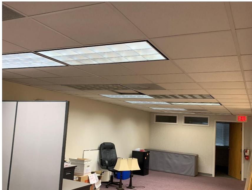
Recessed Fluorescent Lighting in the office Space of the 2 nd Floor Front Mezzanine Area of the Subject Property
