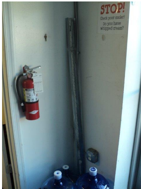
Homogeneous Material No. 6 – Non-ACM White Dry Wall with White Joint Compound located throughout Ben and Jerry Area
