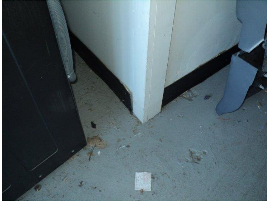
Homogeneous Material No. 7 – Non-ACM Black 4" Vinyl Cove Base with Light Yellow Mastic located throughout Ben and Jerry Area
