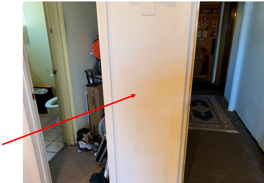
Homogeneous Material No. 8 – Non-ACM White Dry Wall with White Joint Compound located throughout Inner Studio Area
