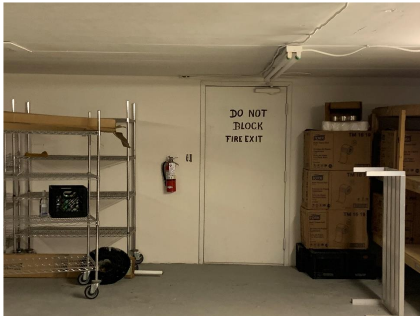
Fire Extinguisher in the Storage Areas of the Subject Property
