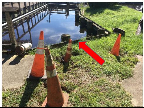
**Photo No. 1 Description:** View of Constitution Park sidewalk looking South. Arrow points to bulkhead sheet piling to be replaced.
