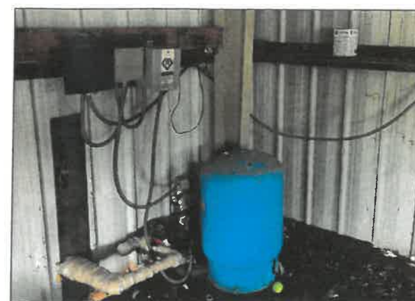
4 EXISTING WELL PUMP SYSTEM
