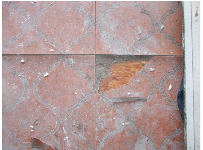
Photo 10 – 12" x 12" brown thin pattern floor tile & adhesive in the main hallway.
