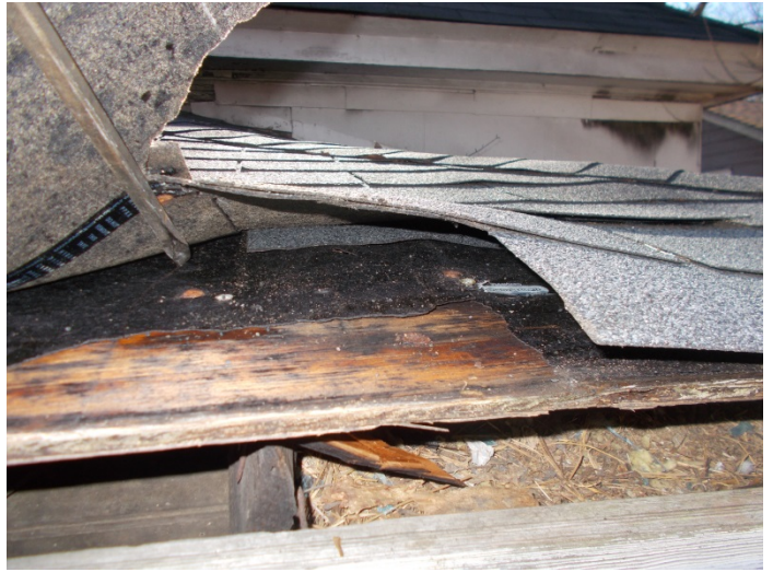
Photo 2 – Roof shingles and felt.
