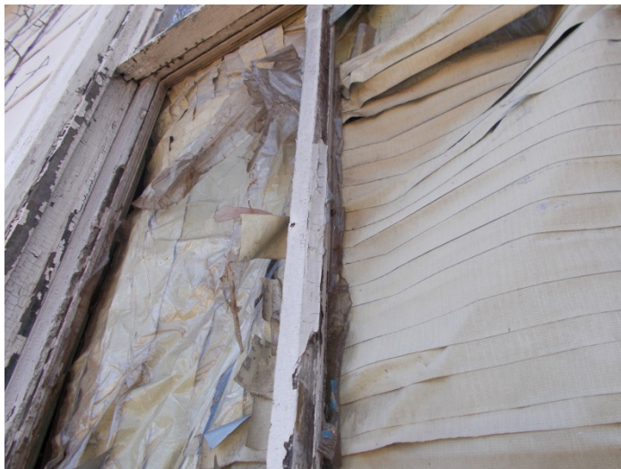
Photo 3 – Wooden windows with glazing.
