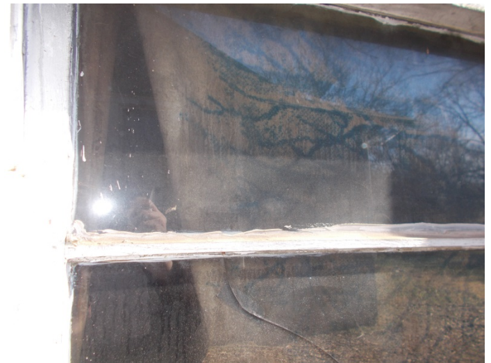
Photo 4 – Wooden windows with caulk.
