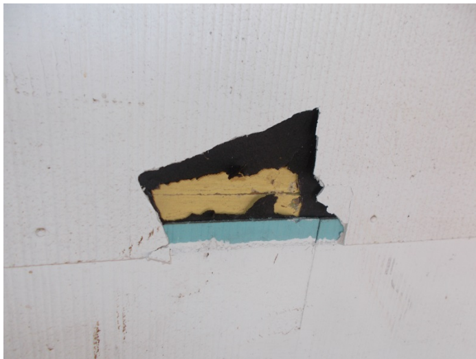
Photo 5 – Cement board siding with felt beneath.
