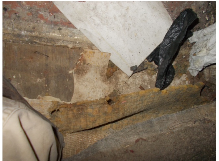
Photo 12 – Yellow pattern vinyl floor with no mastic in the front right bedroom under carpet.
