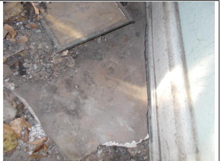
Photo 14 – Brown pattern vinyl floor with no mastic in the kitchen (top layer).
