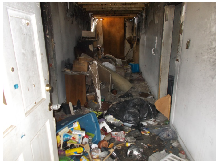
Photo 18 – Typical view inside.
