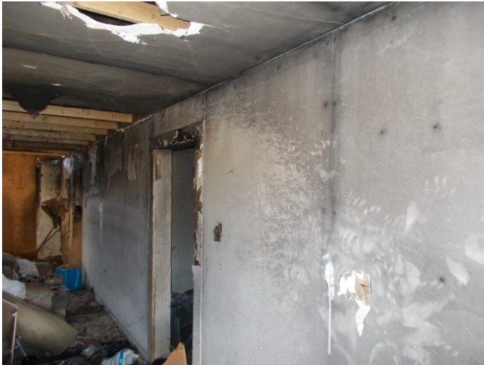
Photo 7 – Drywall with joint compound & tape.
