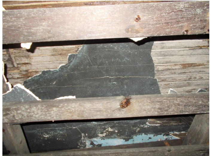
Photo 8 – Plaster with finish.
