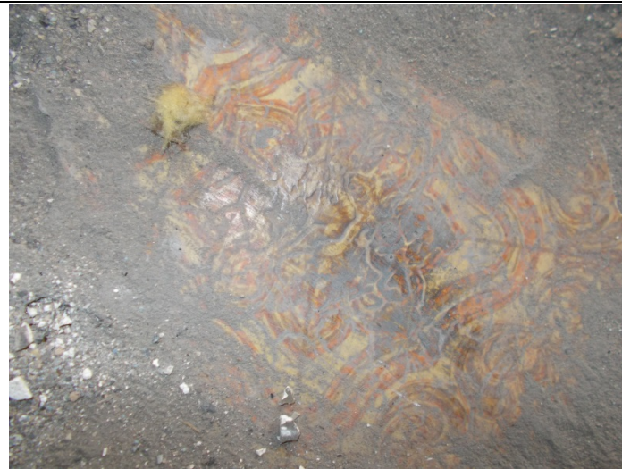
Photo 13 – Beige paisley pattern vinyl floor with no mastic in the dining room in front of the kitchen.
