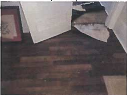
HOMOGENEOUS AREA 23 VINYL SHEET FLOORING (DARK WOOD)
