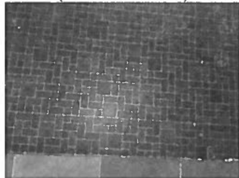
HOMOGENEOUS AREAS 17, 18 VINYL SHEET FLOORING (BLUE BRICK) MASTIC (TAN)
