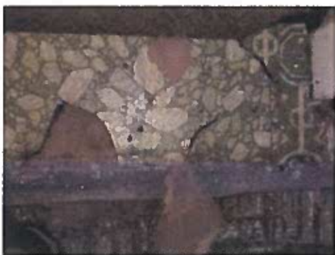
HOMOGENEOUS AREA 23 VINYL SHEET FLOORING (GREEN ROCKS)
