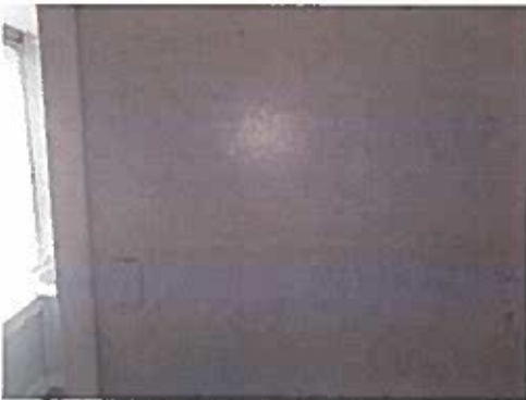
HOMOGENEOUS AREA 09 DRYWALL
