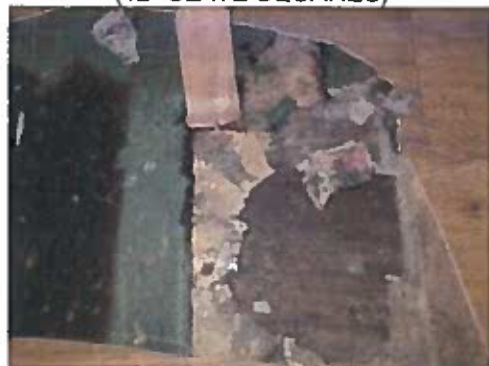
HOMOGENEOUS AREA 18 VINYL SHEET FLOORING (BEIGE/GREEN)
