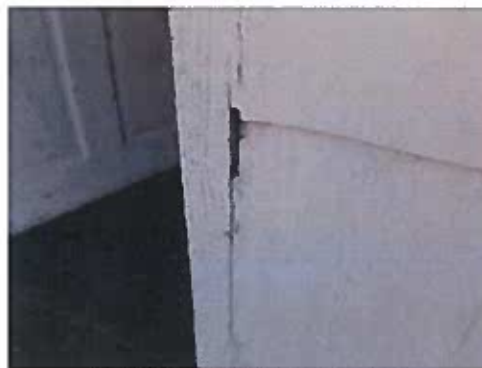
HOMOGENEOUS AREA 04 EXTERIOR CAULK
