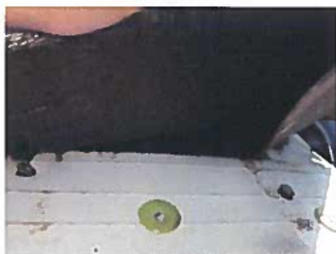
HOMOGENEOUS AREA 06 ROOF FELT
