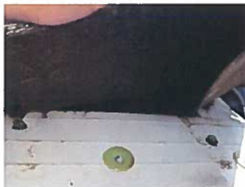
HOMOGENEOUS AREA 06 ROOF FELT
