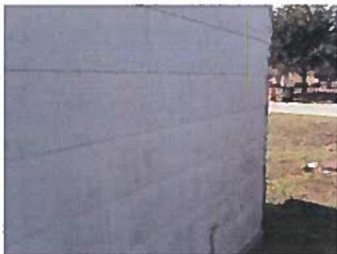
HOMOGENEOUS AREA 01 TRANSITE SIDING
