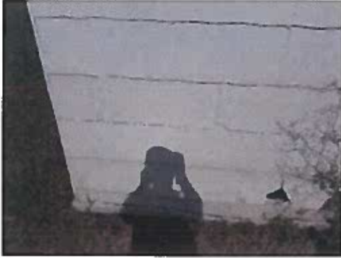
HOMOGENEOUS AREA 01 TRANSITE PANEL
