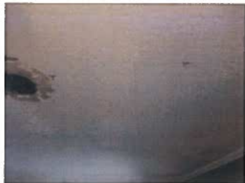
HOMOGENEOUS AREA 12 CEILING TEXTURE (STAPLED)
