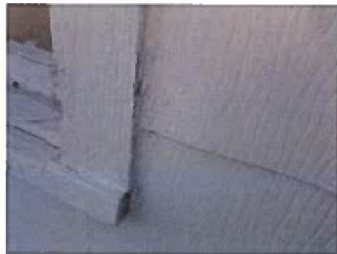
HOMOGENEOUS AREA 04 EXTERIOR CAULK
