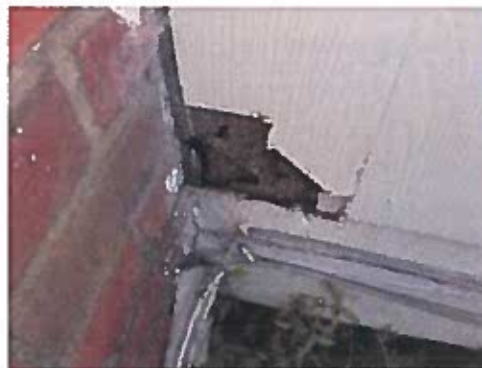
HOMOGENEOUS AREA 02 SIDING FELT
