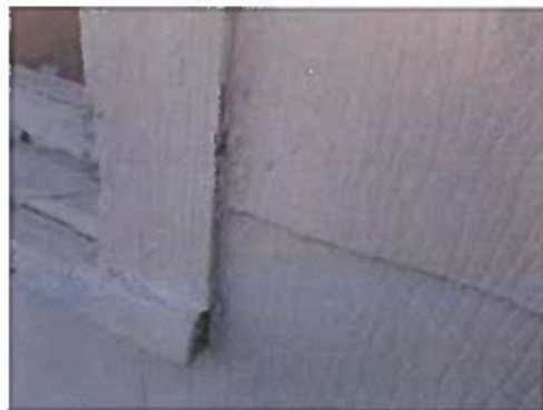
HOMOGENEOUS AREA 04 EXTERIOR CAULK
