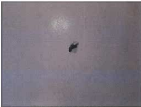
HOMOGENEOUS AREA 09 DRYWALL
