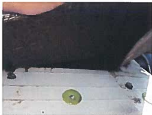
HOMOGENEOUS AREA 06 ROOF FELT
