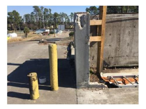
Repair Wall Remove/cut off existing rebar Repair Concrete as per structural drawings and as per Section 03930 Maintenance of Concrete.
