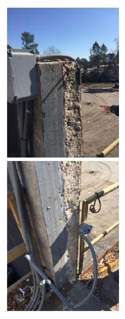
Repair Concrete as per structural drawings and as per Section 03930 Maintenance of Concrete Remove/cut off existing rebar Relocate and reattach electrical conduit
