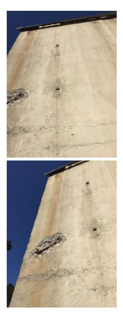
Repair concrete spalling at rebar and holes. Repair Concrete as per structural drawings and as per Section 03930 Maintenance of Concrete
