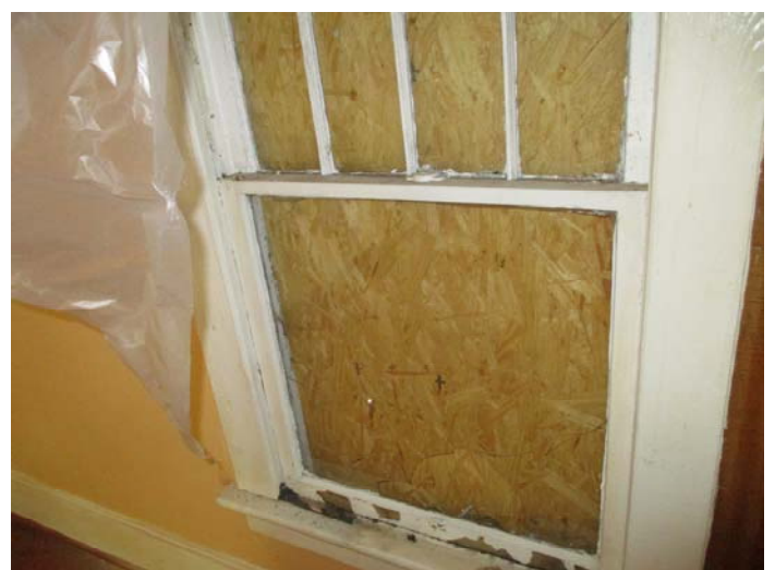
Photo 10 – Wooden windows with glazing
