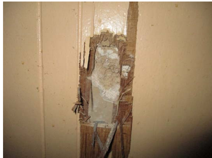
Photo 3 – Plaster & finish walls & ceilings throughout
