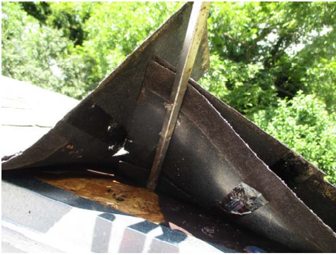
Photo 13 – Roof shingles & felt
