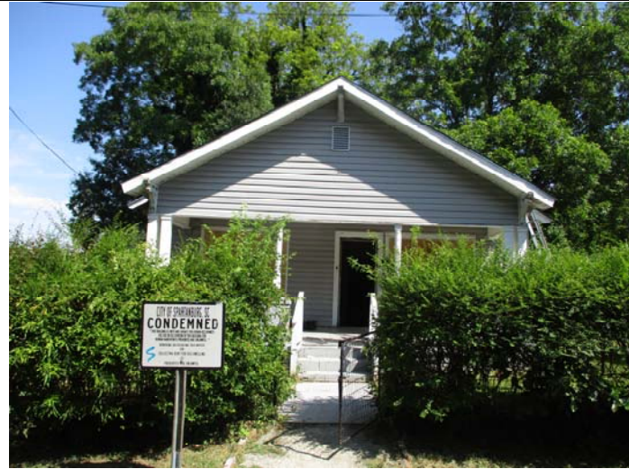
Photo 1 – 418 Carpenter Street in Spartanburg, South Carolina 29301
