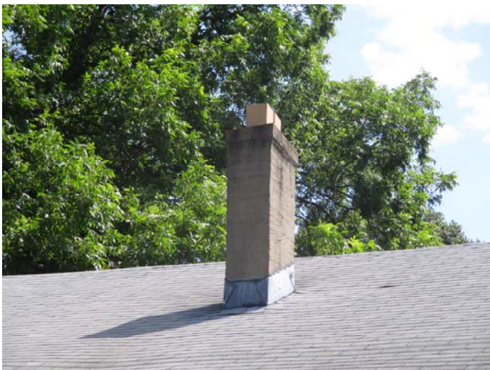
Photo 11 – 1 of 2 chimneys with tar – assumed positive
