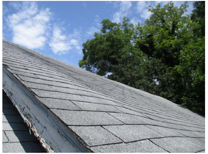
Photo 14 – Roof shingles & felt
