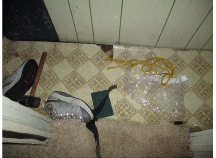
Photo 16 – Tan & brown square pattern roll vinyl floor with no adhesive in the back left bedroom closet
