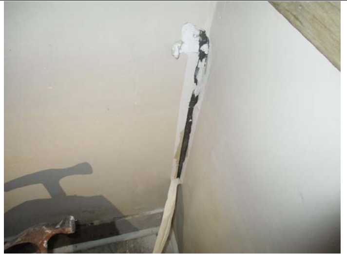
Photo 2 – Drywall with joint compound & tape walls & ceilings throughout
