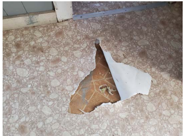
Photo 4 – Two layers of roll vinyl located over wood floors in kitchen, bathroom, bedroom and hallway.
