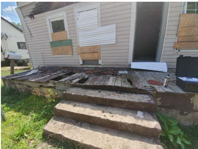
Photo 11 – Rotten wood on front porch is unstable.
