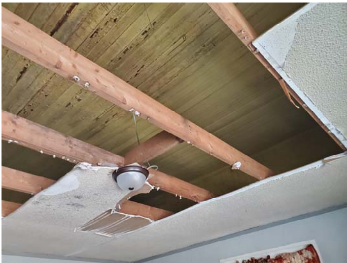
Photo 3 – Textured ceiling over drywall throughout.
