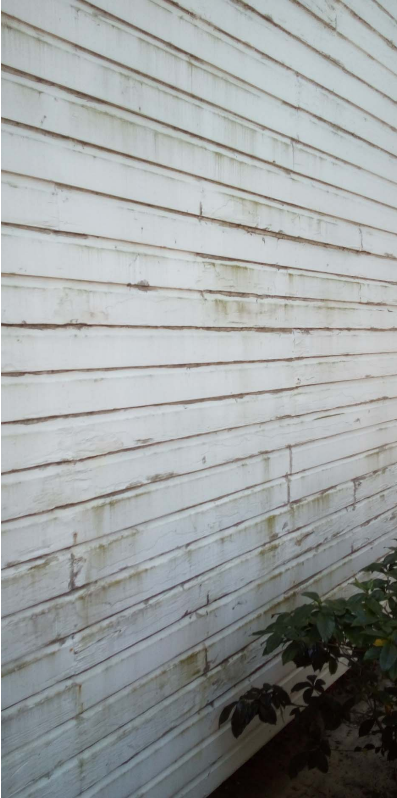
Close up of North wall
