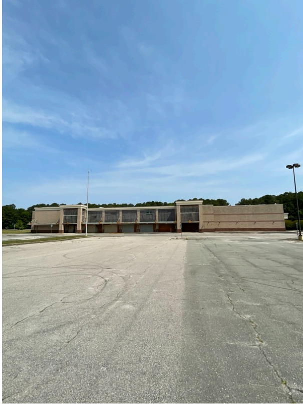
General view of the Former Kroger structure on the Subject Property
