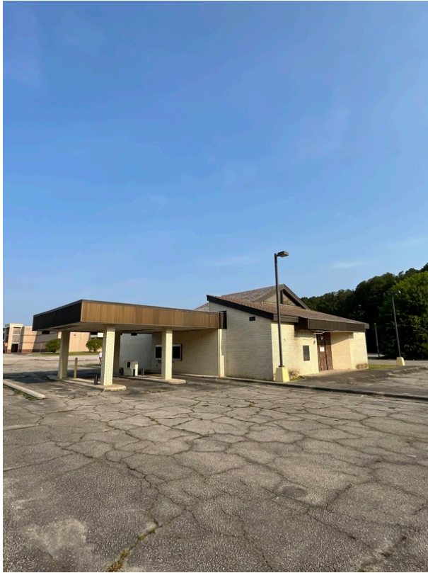
General view of the Former Bank structure on the Subject Property
