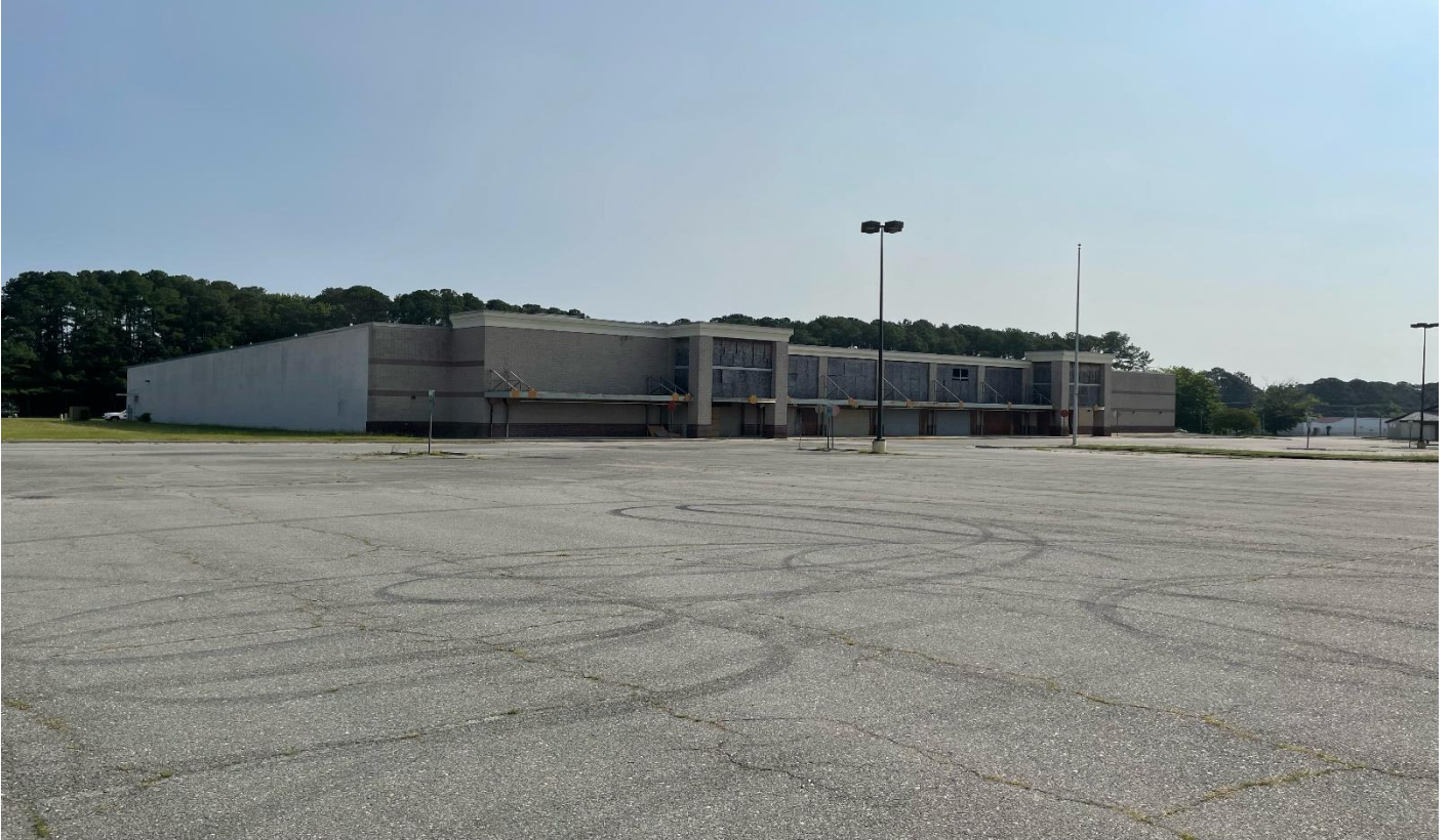
Pictures of buildings to be demolished (former Kroger and bank buildings) (Estimated Square Footages: former Kroger and former bank 60,000 square foot total)
