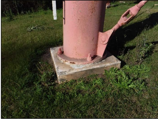
Tank Column Foundation
