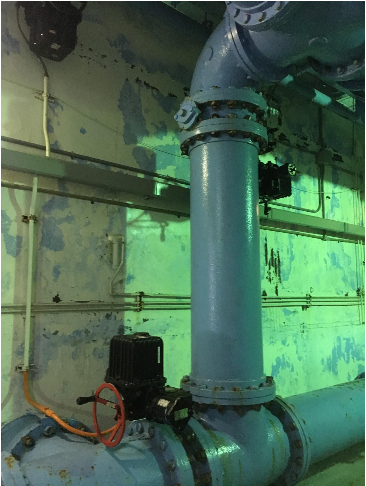
Close-up of Filter Piping and Valves
