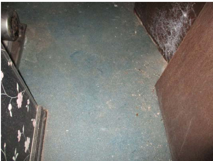
Photo 11 – Blue pattern vinyl floor with no adhesive in the left side 1st bathroom on the right
