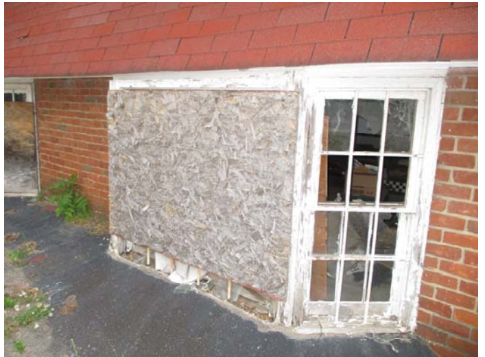
Photo 4 – Wooden window with glazing
