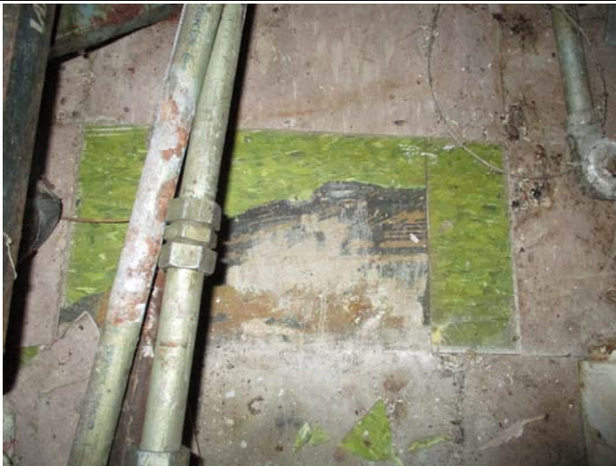
Photo 15 – 2 nd layer 12" x 12" green peacock floor tile & black mastic in the right side 1st room on the right
