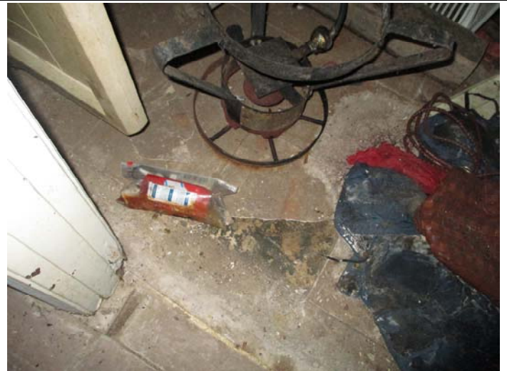
Photo 16 – 12" x 12" floor tile & black mastic in the right side 3rd & 4th rooms on the right
