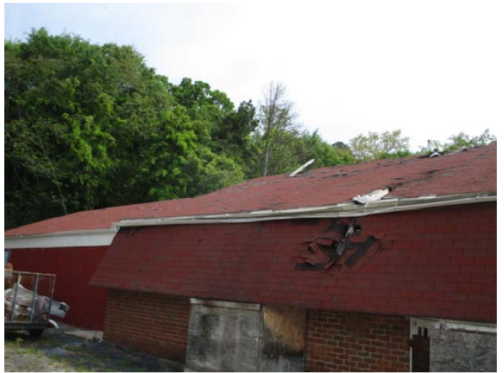
Photo 2 – Roof shingles & felt
