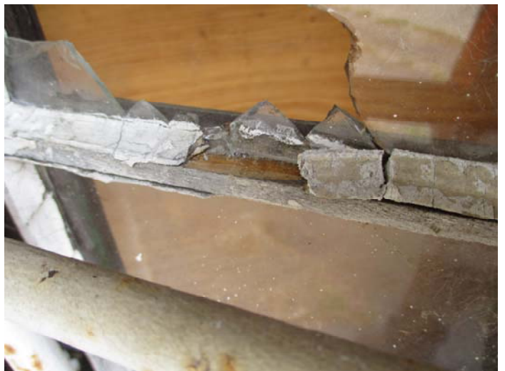
Photo 6 – Wooden window with base, inner & outer layers
