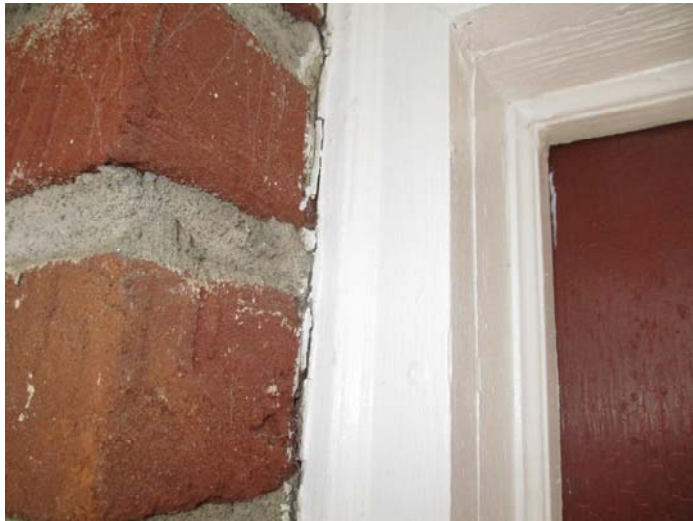
Photo 3 – White wooden door caulk
