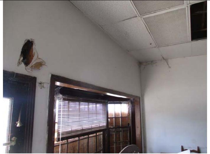
Photo 20 – Drywall with joint compound & tape in the left side walls & bathrooms & throughout the right side except in the back room
