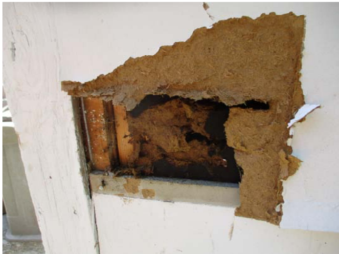
Photo 9 – Felt paper beneath wooden & vinyl siding
