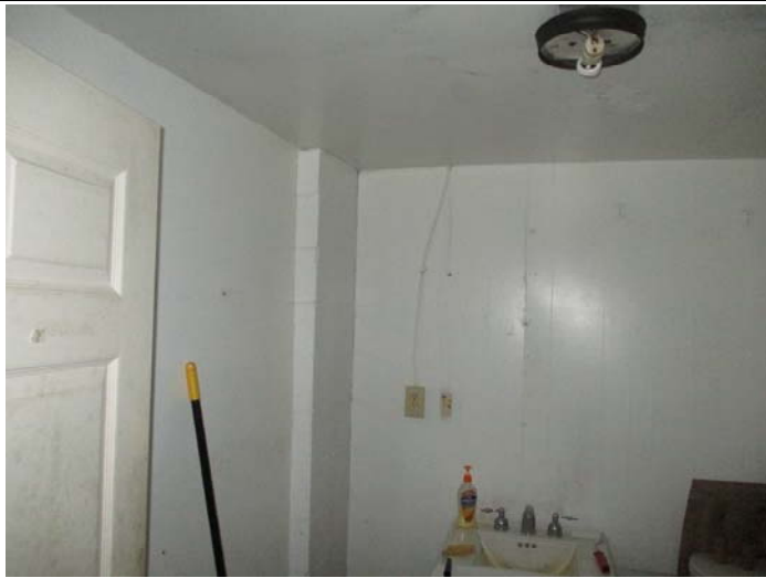
Photo 15 – Typical view of a bathroom and drywall walls & ceilings
