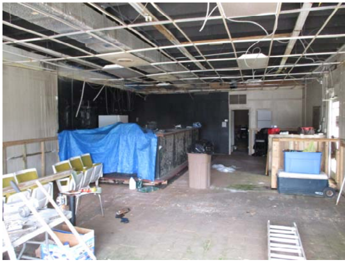
Photo 13 – Typical view of the front area
