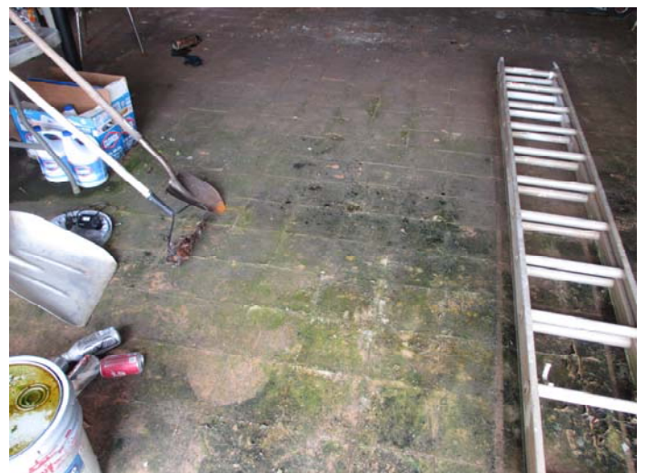
Photo 12 – 9" x 9" brown floor tile & brown mastic in the front area
