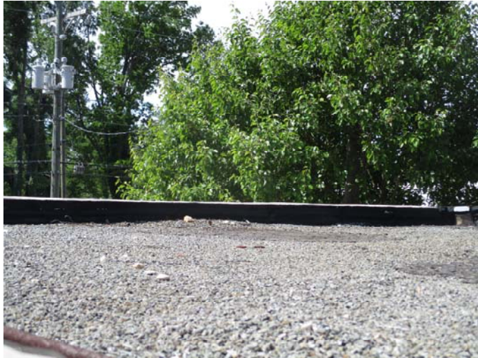
Photo 7 – tar & shingle flashing on the flat roof parapet walls & stone
