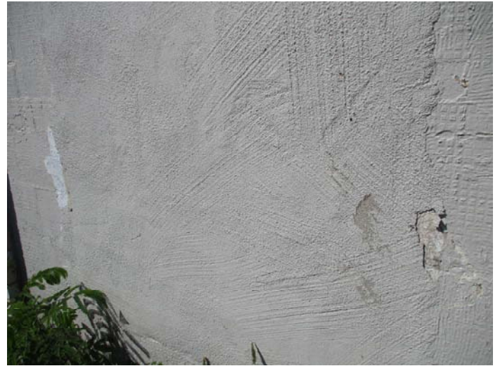
Photo 2 – Stucco over CMU blocks
