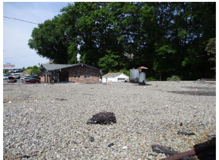
Photo 6 – Built up tar and gravel roof system
