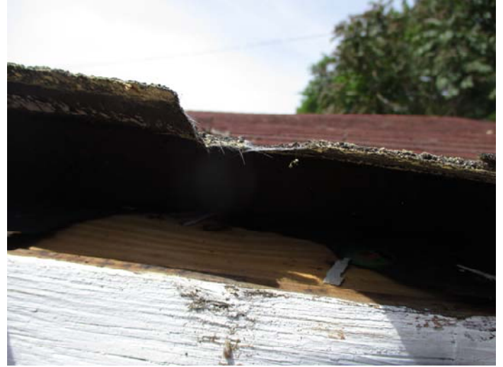
Photo 8 – Roof shingles & felt on back pitched wooden roof
