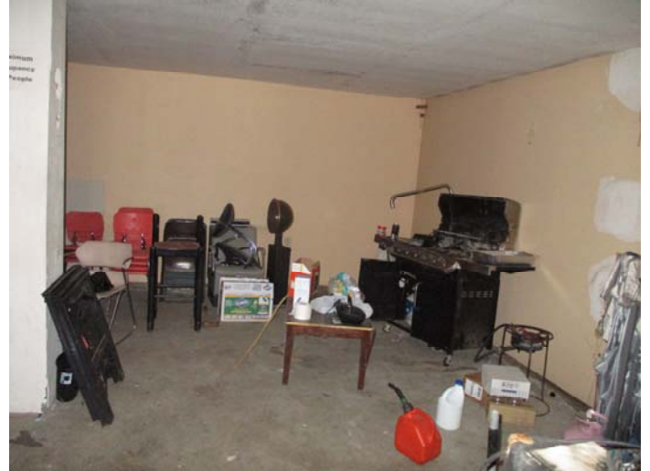
Photo 14 – Typical view of the back area and drywall walls & ceilings
