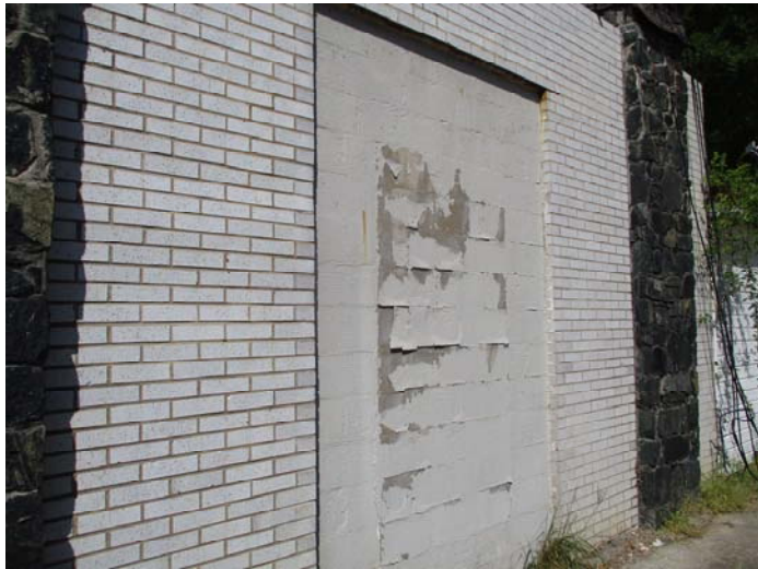
Photo 3 – Stucco over CMU blocks
