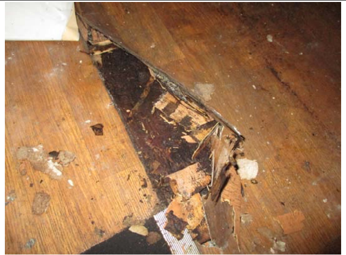
Photo 16 – Multiple layers of roll vinyl flooring & adhesives behind the bar area
