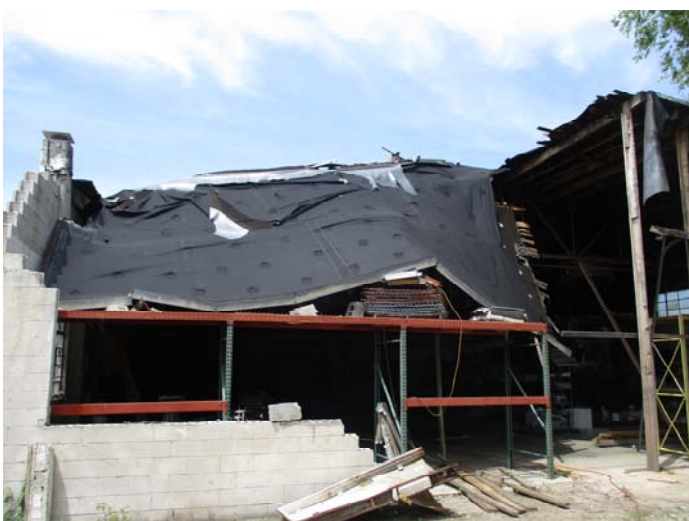
Photo 11 – Roof felt & rubber membrane on back warehouse roof
