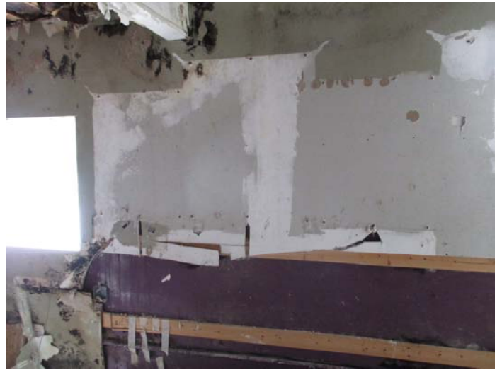
Photo 14 – Drywall with joint compound
