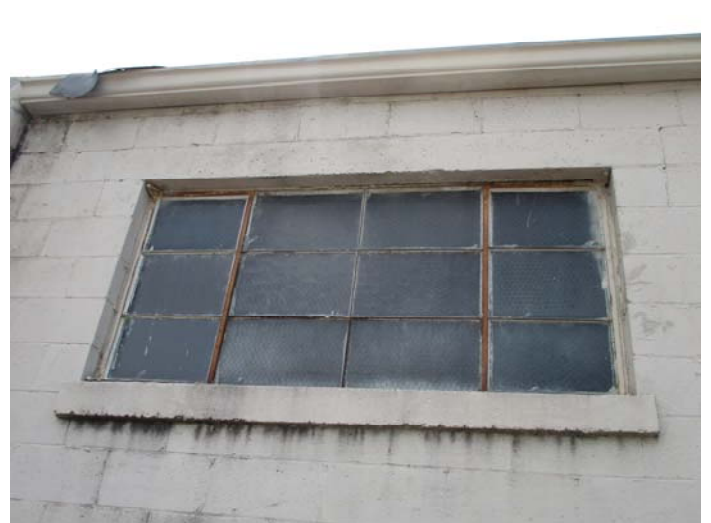
Photo 6 – Back metal window with glazing
