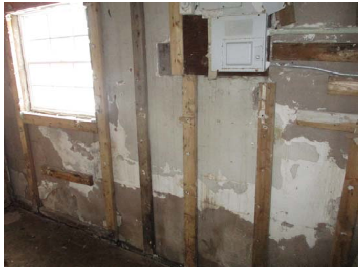
Photo 16 – Plaster with finish walls
