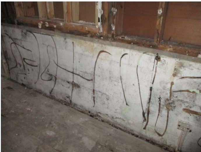
Photo 17 – Wall panel adhesive in the front area
