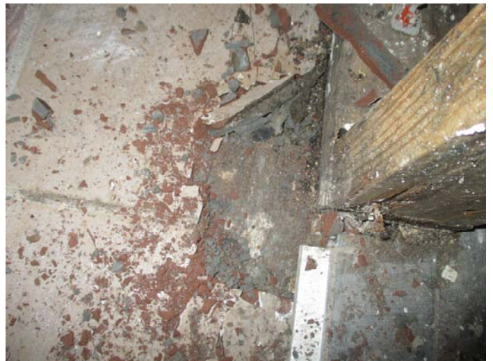
Photo 18 – Gray leveling compound in the front area
