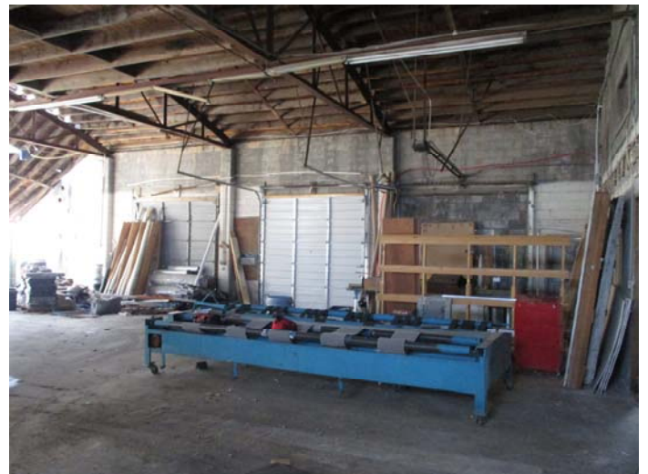
Photo 24 – Typical view of the back warehouse area
