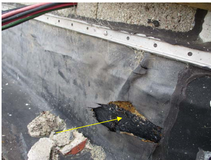
Photo 5 – Flashing tar on the flat roof
