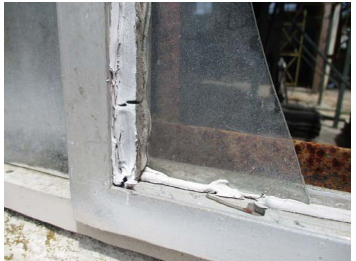
Photo 10 – Caulk patch on back metal windows
