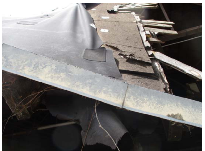
Photo 12 – Roof felt & rubber membrane on back warehouse roof
