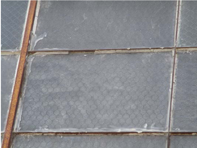
Photo 7 – Back metal window with glazing
