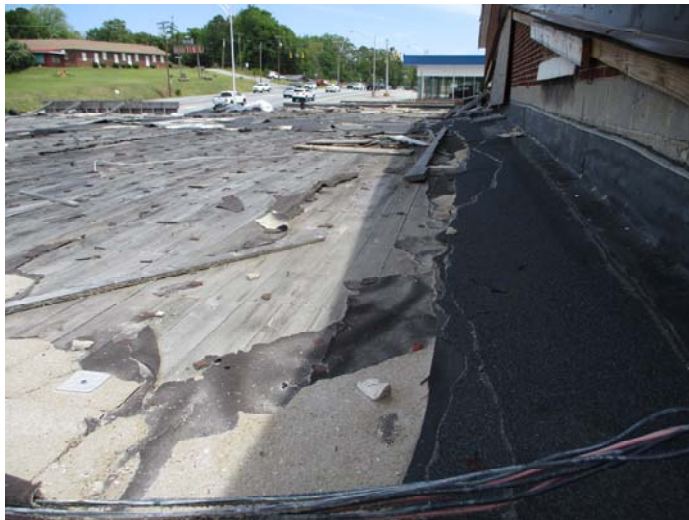
Photo 3 – Roll roofing over brown insulation & felt paper on the front roof
