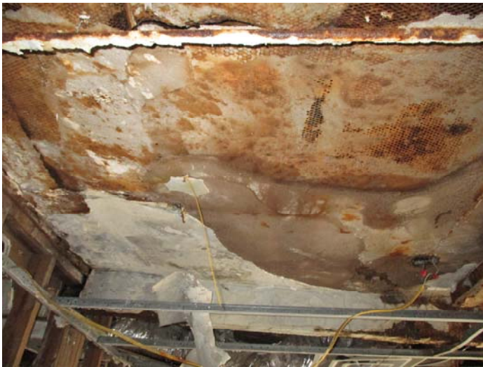
Photo 15 – Plaster with finish ceilings
