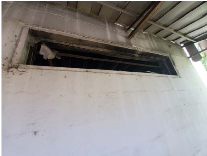
Photo 3 – Front metal window with glazing
