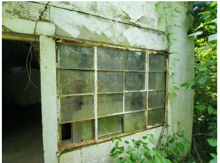
Photo 4 – First floor back metal window with glazing
