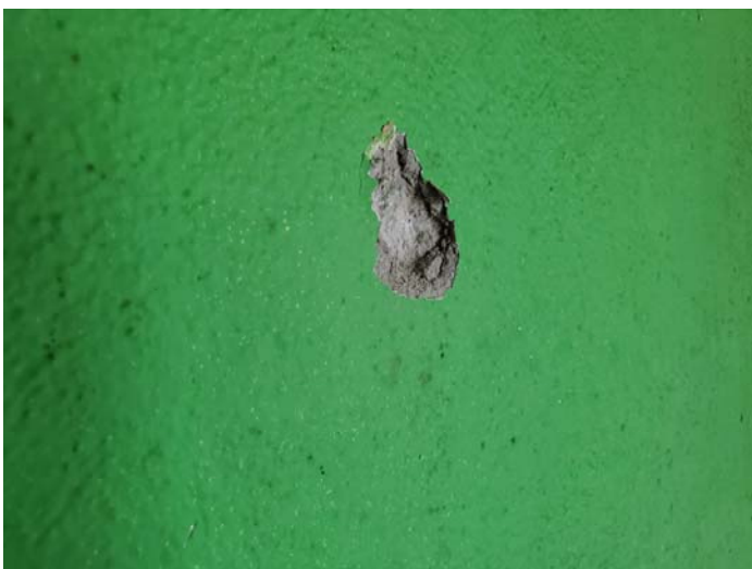
Photo 11 – Skim coat over CMU block wall located in section A/B.
