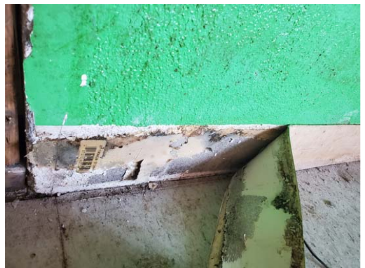
Photo 12 – Tan mastic under cove base located in section A/B
