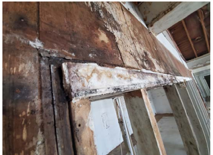
Photo 22 – Drywall, joint compound and tape on walls sporadic in section A/B
