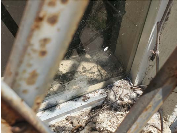
Photo 7 – Close up of 706C metal window with white caulk
