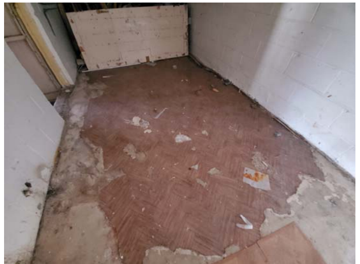
Photo 16 – Wood pattern roll vinyl floor located in section C hallway
