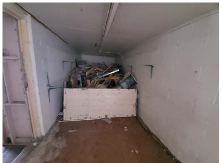
Photo 24 – Various types of building debris stacked in back hallway of section C
