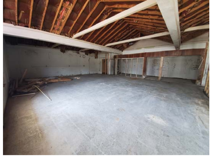
Photo 8 – Interior view of back portion of 706A/B
