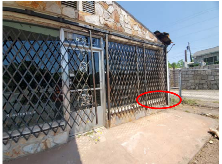
Photo 6 – 706C metal window with white caulk
