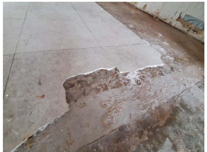
Photo 10 – 12"x12" white with gray/blue specks floor tile with tan adhesive
