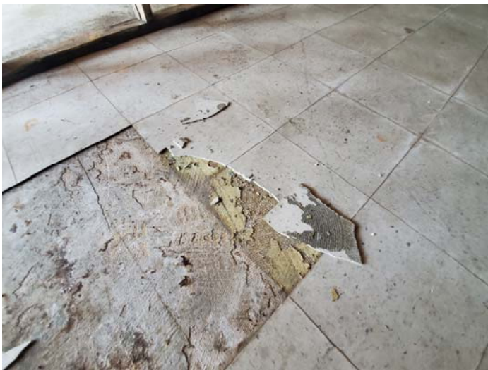
Photo 9 – 12"x12" white with gray/blue specks floor tile with gray and tan mastic located in section A/B
