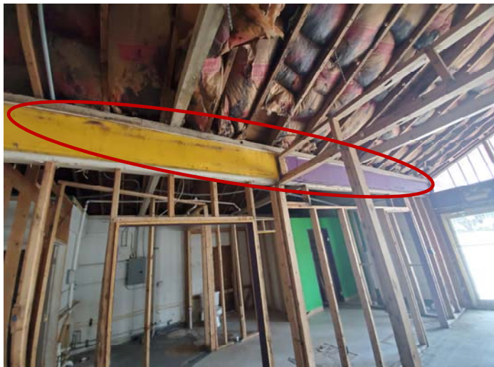
Photo 21 – Joint compound skim coat over ceiling beams located in section A/B
