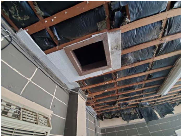
Photo 19 – 12"x12" white ceiling tiles without mastic located in section C
