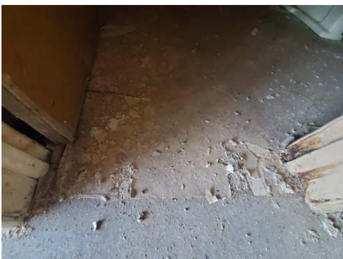
Photo 17 – Tan rock pattern roll vinyl flooring located in section C bathroom
