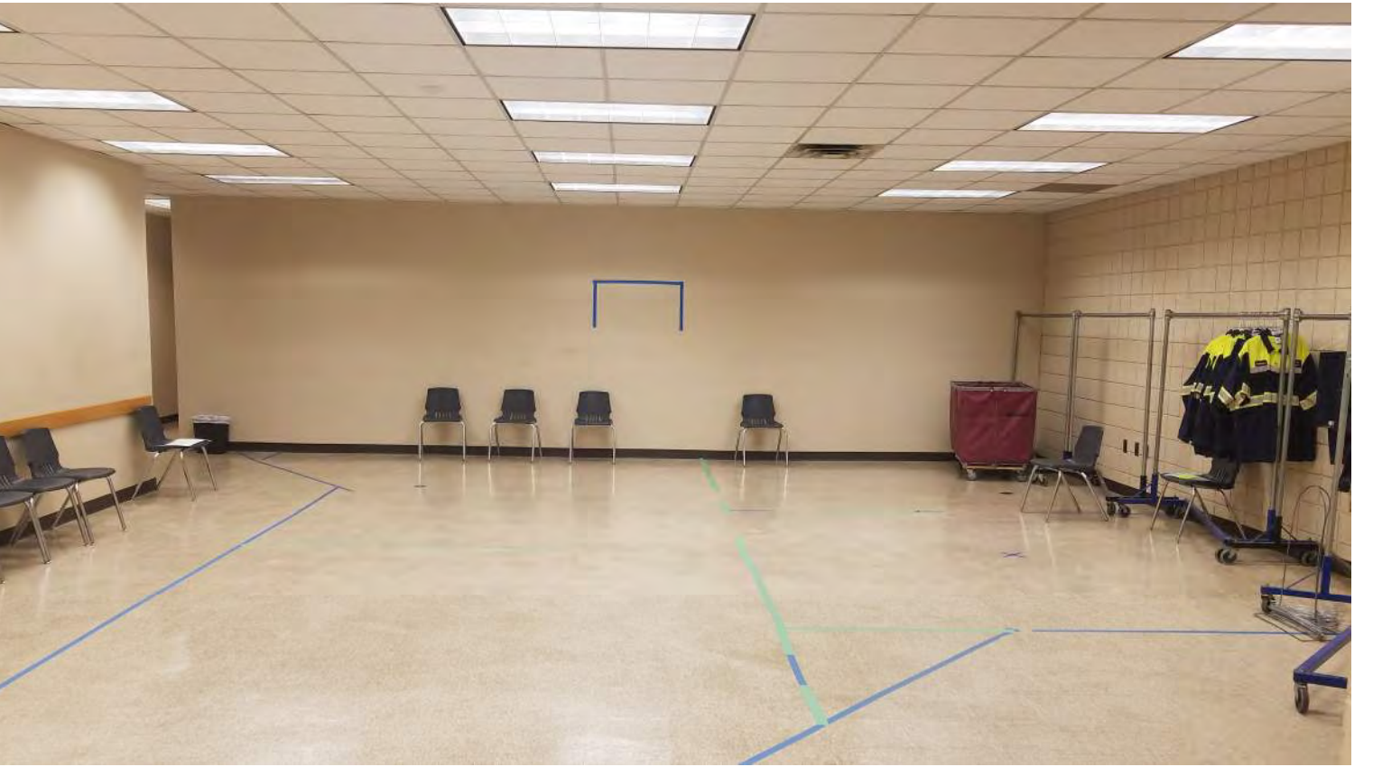
4 PHOTO NOT TO SCALE B-1 EXISTING CONDITIONS
