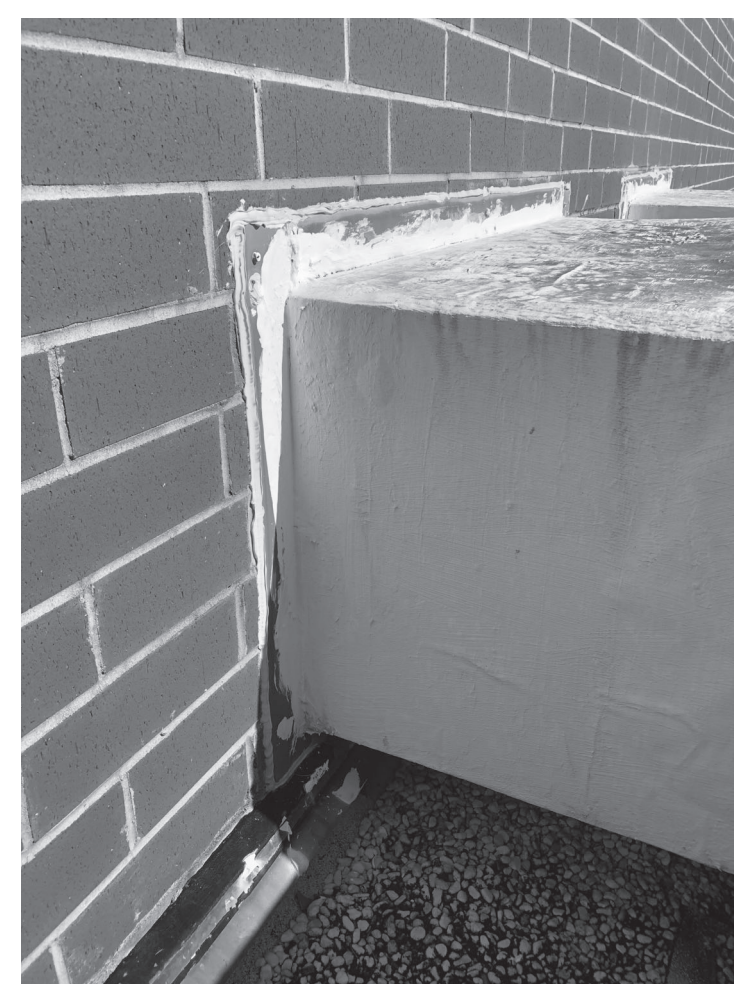
C RETURN DUCT @ EXTERIOR WALL 1/2" = 1'-0"
