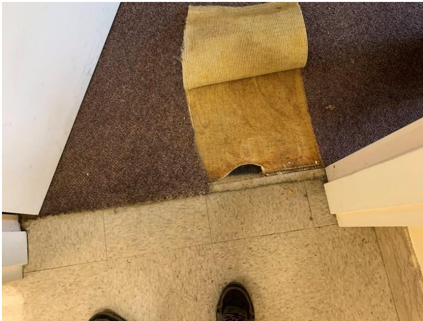
Homogeneous Material No. 10 – ACM Gray Pebble Pattern Resilient Sheet Flooring over Brown Vinyl Floor tiling with black mastic located in Building Main Floor, Corridor near Elevator
