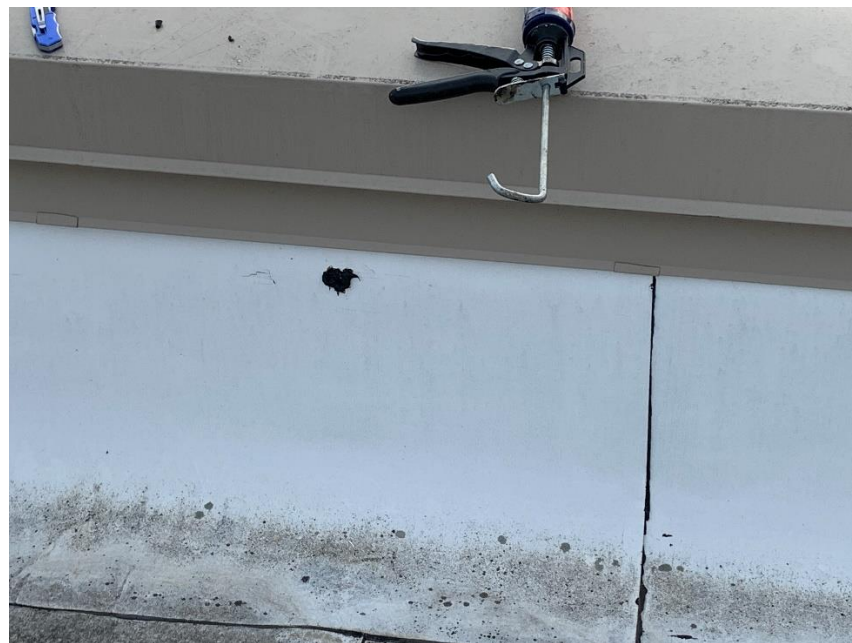
Homogeneous Material No. 2 – Non-ACM White/Black Curbing/Flashing located on the roof of the Subject Property
