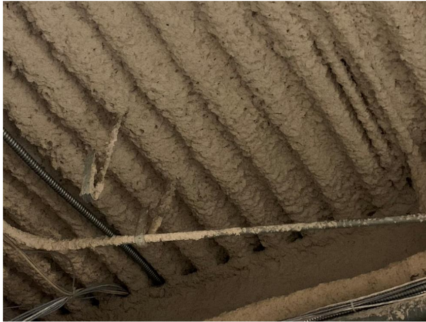
Homogeneous Material No. 5 – Non-ACM Gray Spray-on Fire Proofing located in the Building Basement Corridor, Electrical Room and Boiler Room of the Subject Property
