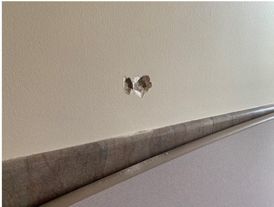
Homogeneous Material No. 11 – Non-ACM Plaster Gray Base White Skim Coat on Wall located in Building Main Floor, Corridor near Elevator of the Subject Property
