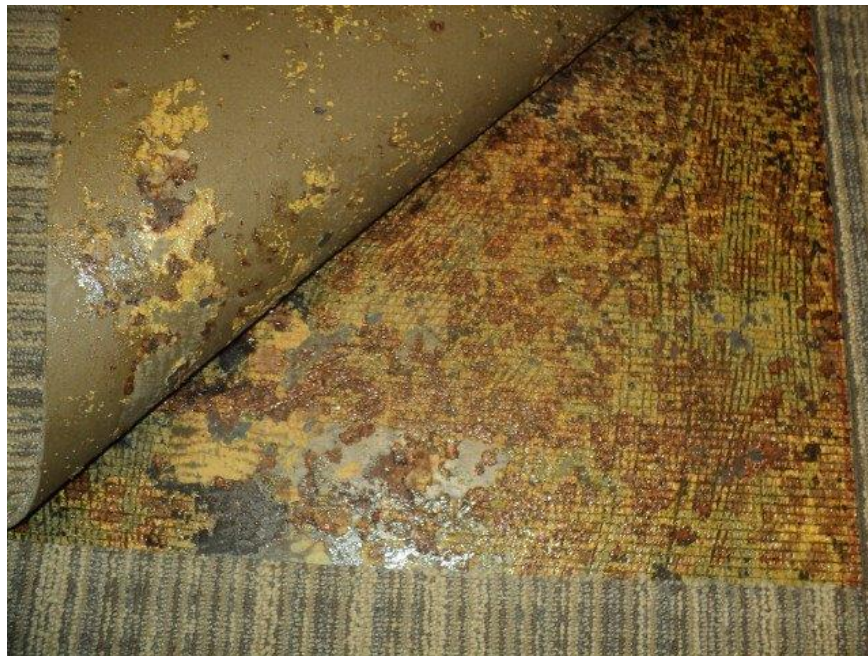
Homogeneous Material No. 16 – Non-ACM Brown/Tan/Black Floor Mastic located in the Building Main Floor, Main Customer Area of the Subject Property
