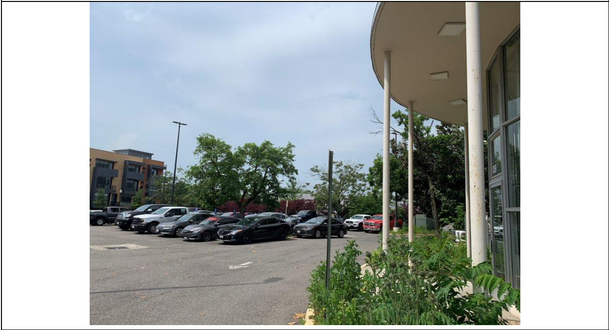
View of the columns and I-Beams at the building rear entrance.
