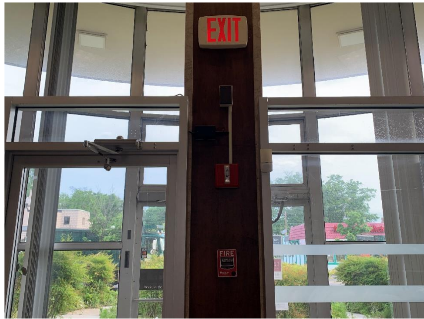
Typical Lighted Exit sign and Fire Emergency Pull-Down station at the subject property building.
