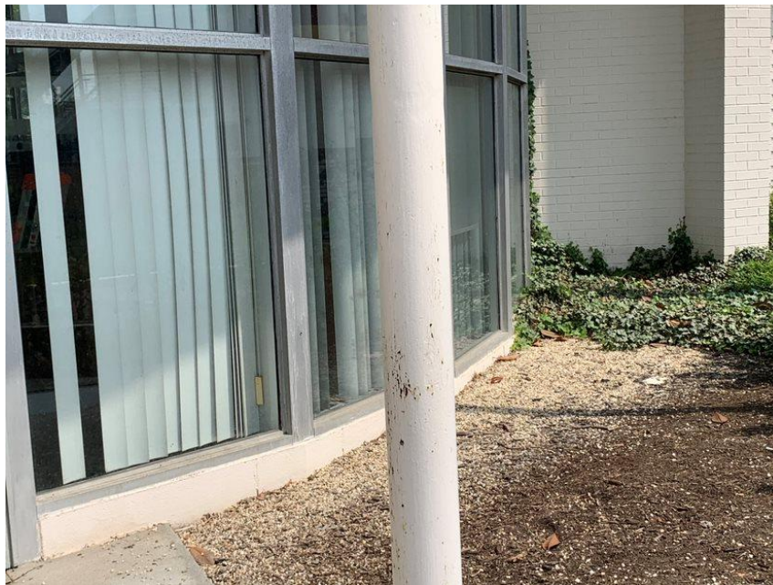
Lead-Containing Paint on the White metal column at the building rear and front entrance.
