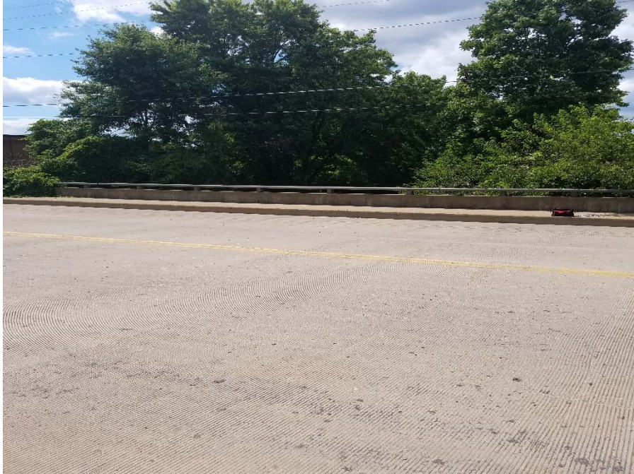
Photo 3 – Wearing Surface & South Sidewalk
