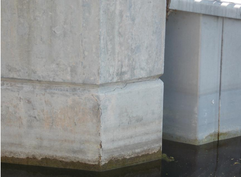
Upstream - East Structure Wall. Note Crack at Construction Joint.
