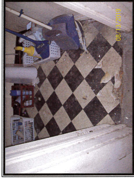
Photo #4 Parquet Sheet Flooring under non-asbestos containing Checkerboard Sheeting in BR 2
