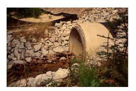
ii. For all exposed crossline pipe ends, when an end treatment is not specified in the plans, use **Pipe Riprap Protection** (804–3xx–xx). For flexible pipe larger than 24" diameter, install pipe straight headwall, pipe end structure, flared end section, or wingwall section in addition to riprap. For all exposed driveway pipe ends where no end treatment is specified in the plans, use **Pipe Riprap Protection** (804–3xx–xx) unless directed otherwise by the engineer.
