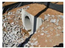
iv. Use **Pipe Straight Headwall** (719–605–00) when specified in the plans or special provisions. Use straight headwall only in locations where pipe exposed end does not face the direction of traffic.
