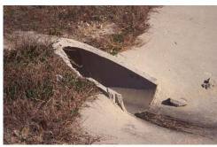
iii. Use **Beveling of Pipe End** (719–610–00) when specified in the plans or special provisions. Beveled ends may only be used on flexible pipe up to 24" diameter and on rigid pipe up to 60" diameter. When beveling of pipe ends is specified on flexible pipe larger than 24" diameter, install pipe straight headwall, pipe end structure, flared end section, or wingwall section. Use factory fabricated beveled ends for all pipe types unless approved by the Engineer.
