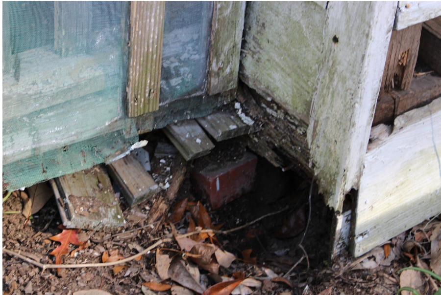
3.2a Foundation System: Dry-Stack Bricks Beneath House
