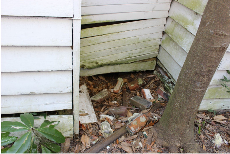
3.2b Perimeter Foundation Drainage: Drainage Problem Where Both Structures Meet
