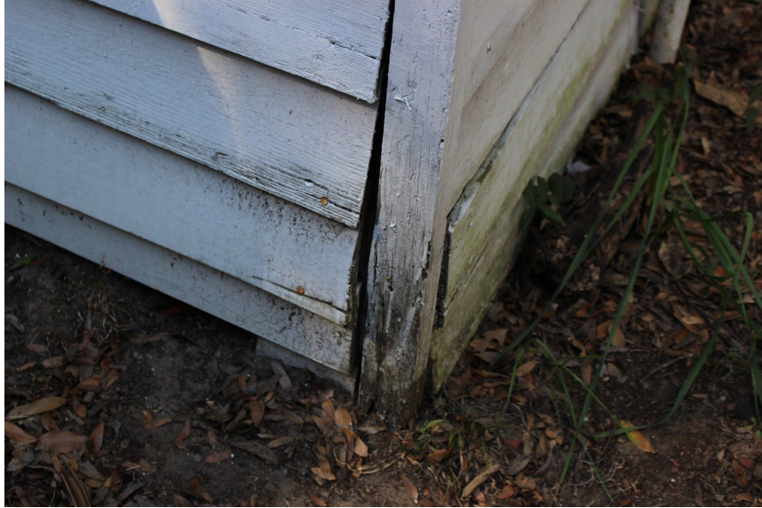
3.2a Foundation System: Wood Posts Sitting Directly on Soil
