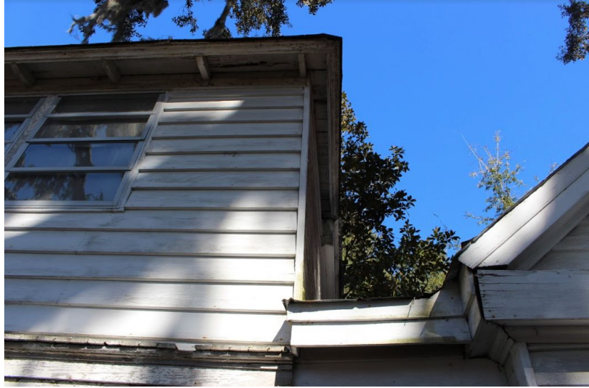
3.5c Drainage System, Gutters, Downspouts: No sign of gutters
