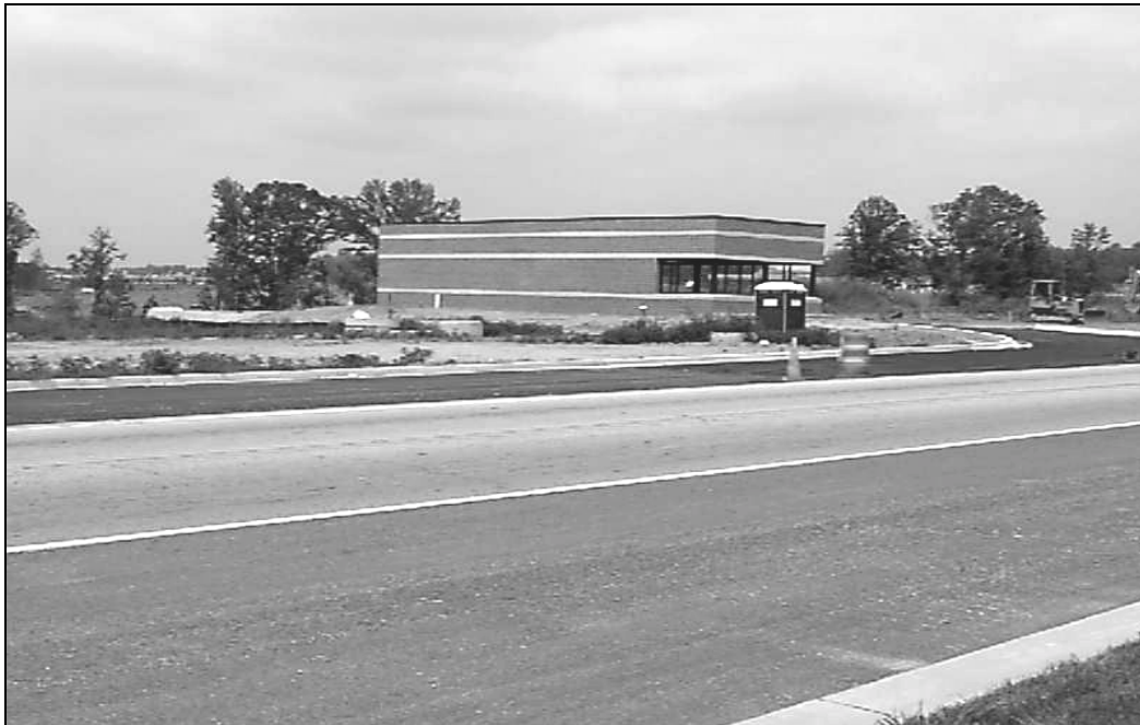
Waffle House under construction on the south side of SR 53 east of Georgia 400
