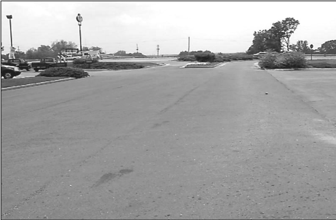
The Dawson 400 shopping center's frontage on the west side of Ga. 400
