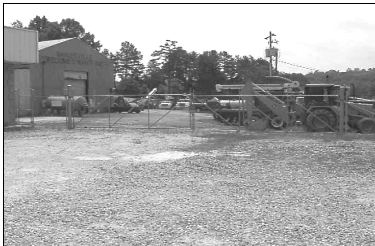
Gainesville Welding and Maintenance, Henry Grady Highway
