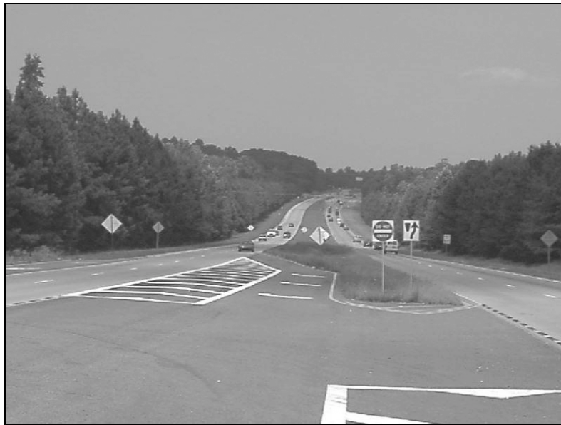
GA 400 North, north of commercial center at intersection of SR 53
