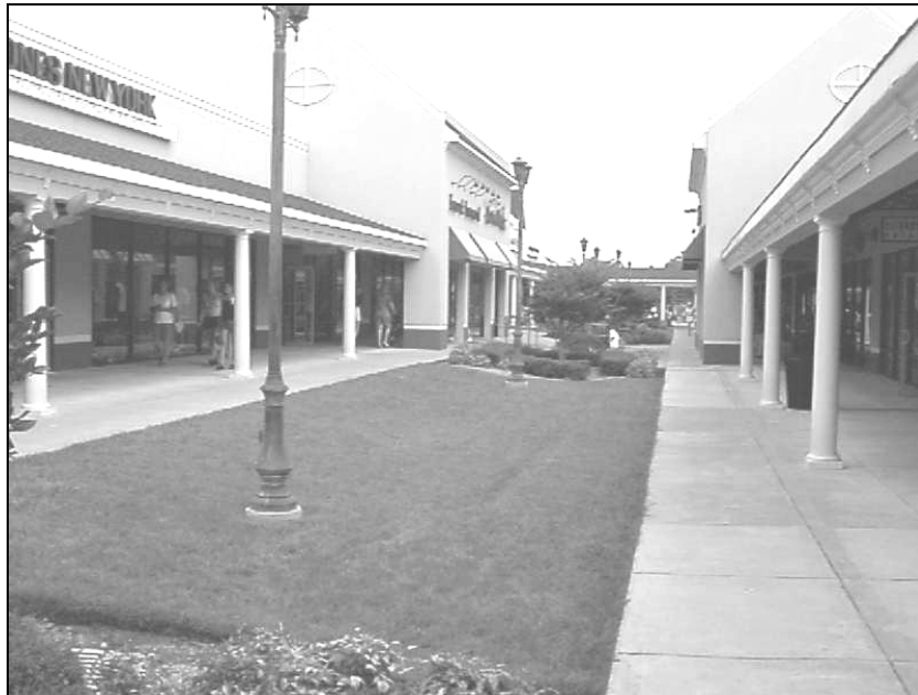
Pedestrian Corridor at North Georgia Premium Outlets
