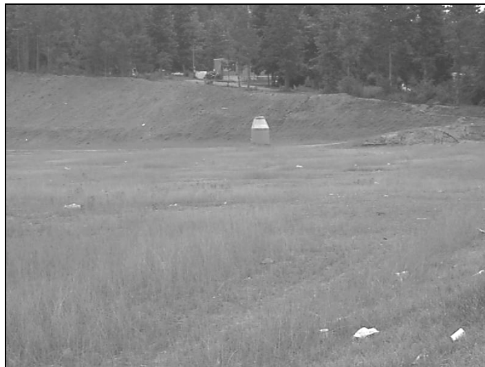
Graded site adjacent to Kroger Shopping Center
