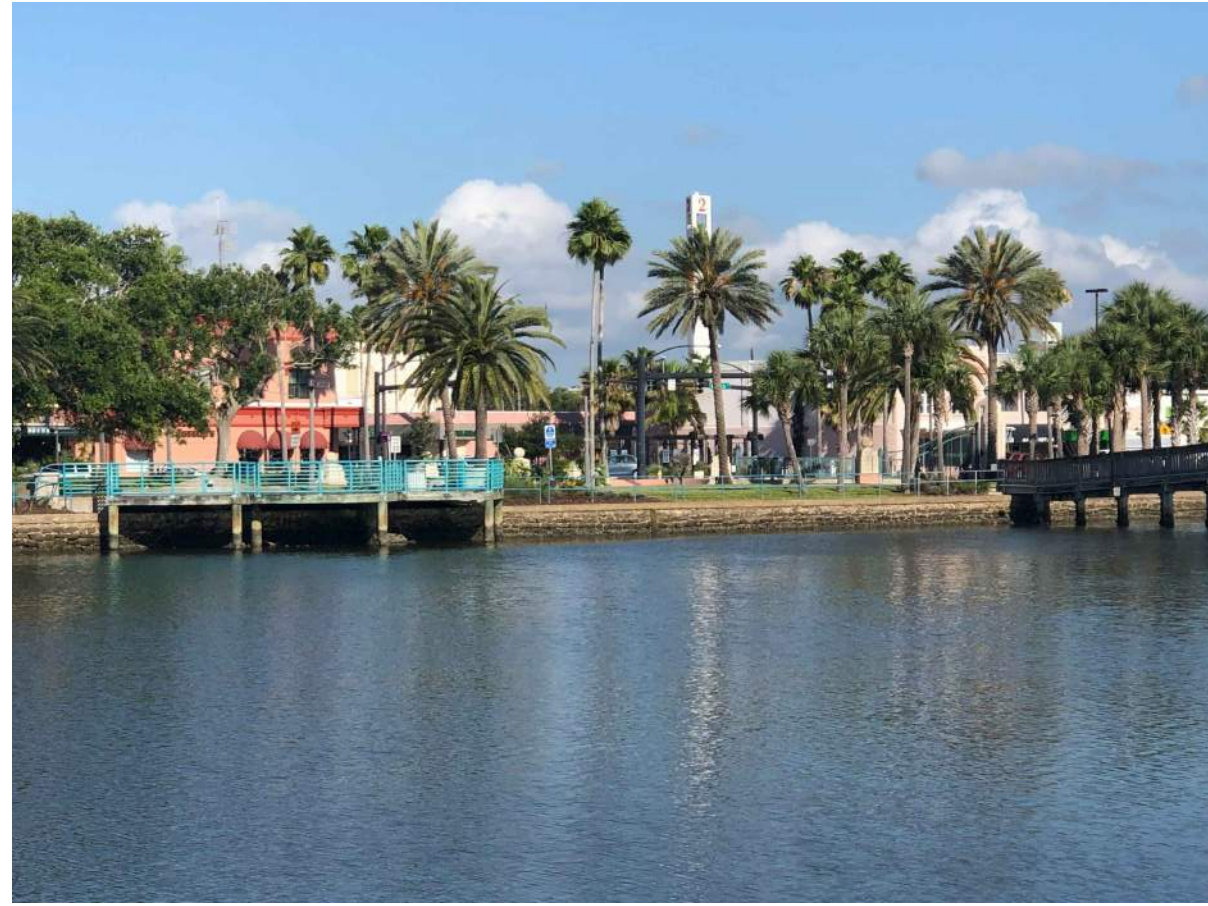
EXISTING BULKHEAD SOUTH OF THE TIMBER BOARDWALK DMC, 2019
