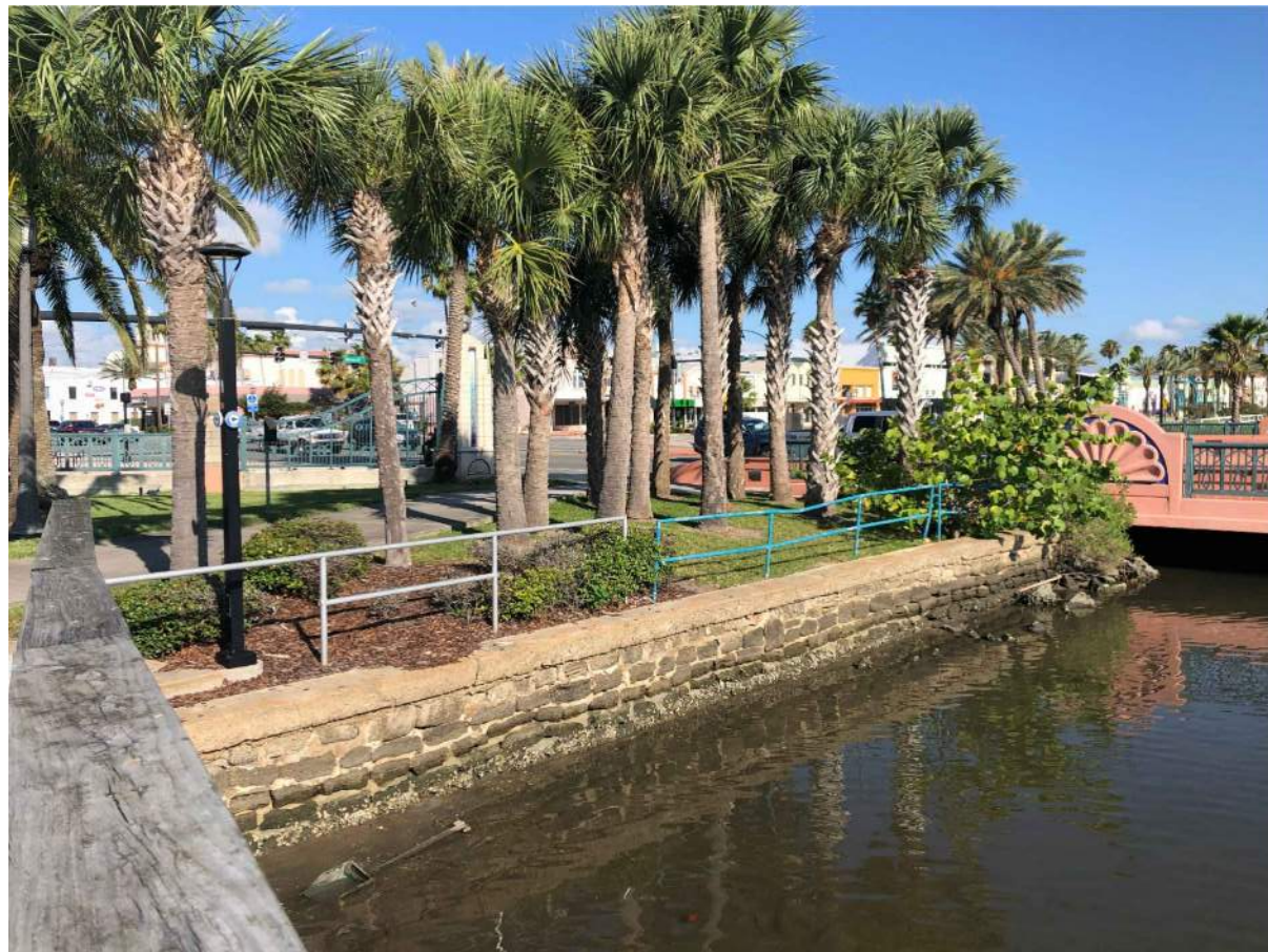
EXISTING BULKHEAD AT INTERNATIONAL SPEEDWAY BOULEVARD DMC, 2019
