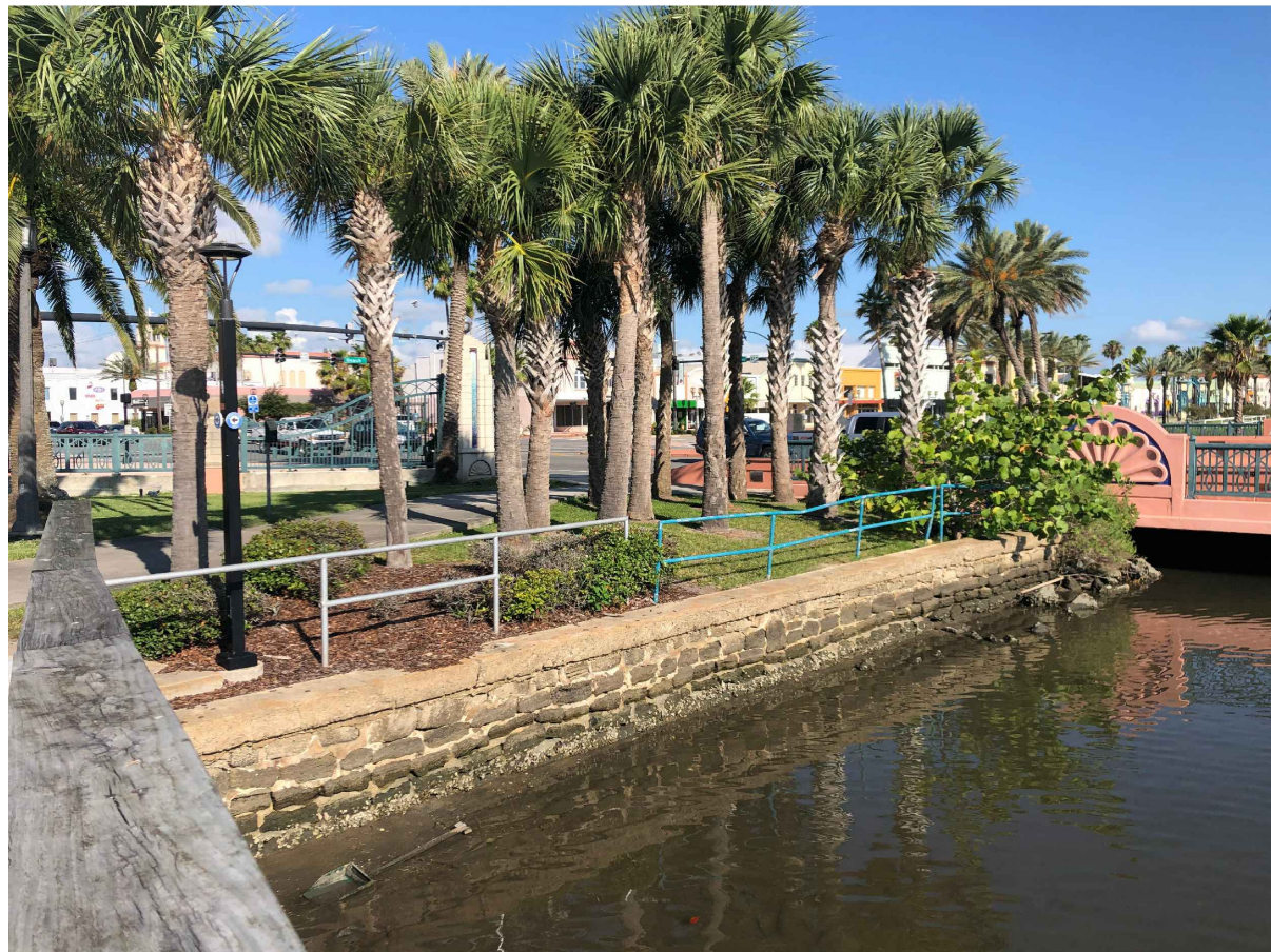
EXISTING BULKHEAD AT INTERNATIONAL SPEEDWAY BOULEVARD DMC, 05.23.2019
