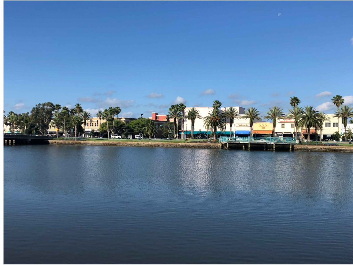
EXISTING BULKHEAD NORTH OF MAGNOLIA AVENUE DMC, 05.23.2019
