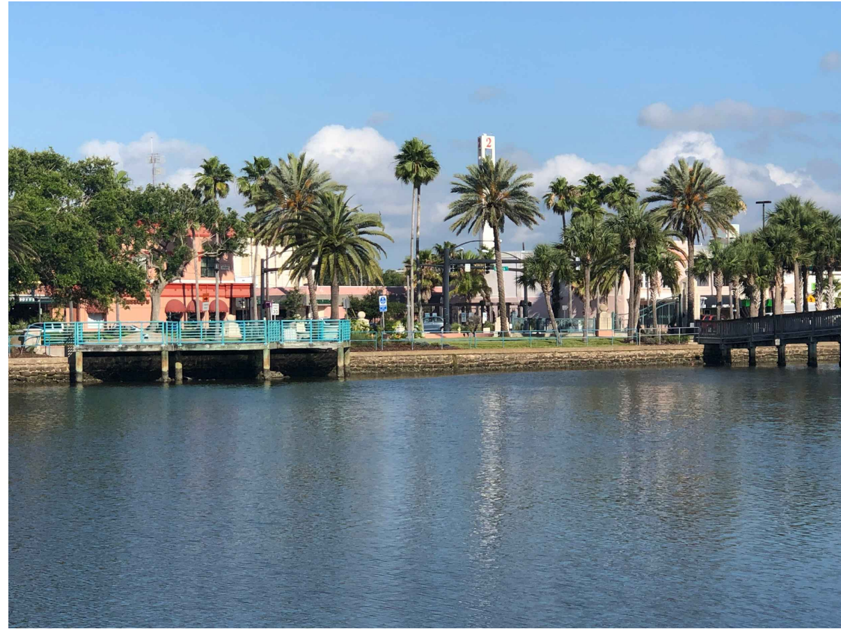
EXISTING BULKHEAD SOUTH OF THE EXISTING PEDESTRIAN BRIDGE DMC, 05.23.2019
