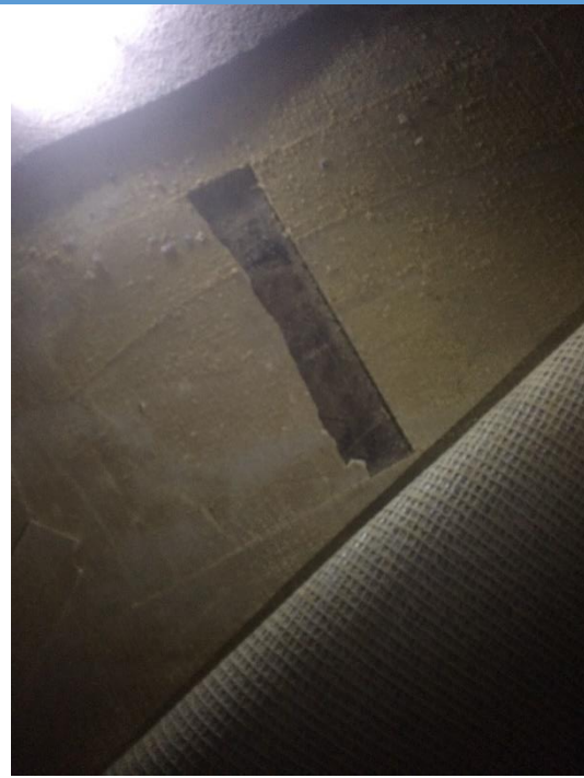
Floor tile under carpet in office areas
