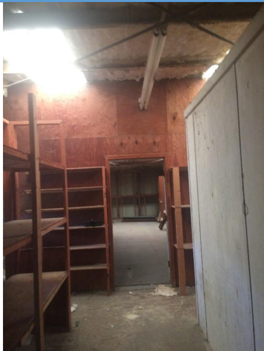
2 nd floor above offices
