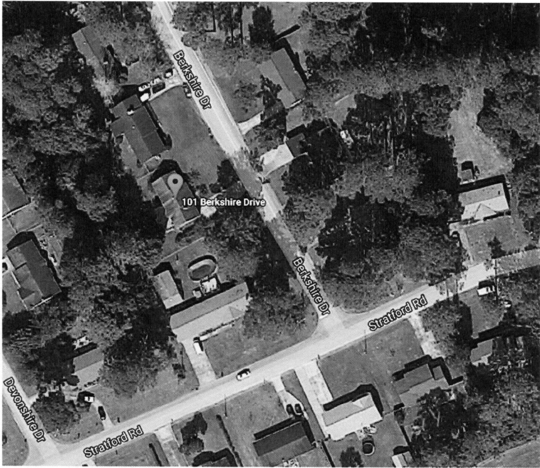
Leaking Fire Hydrant #510, at or near 101 Berkshire Drive
