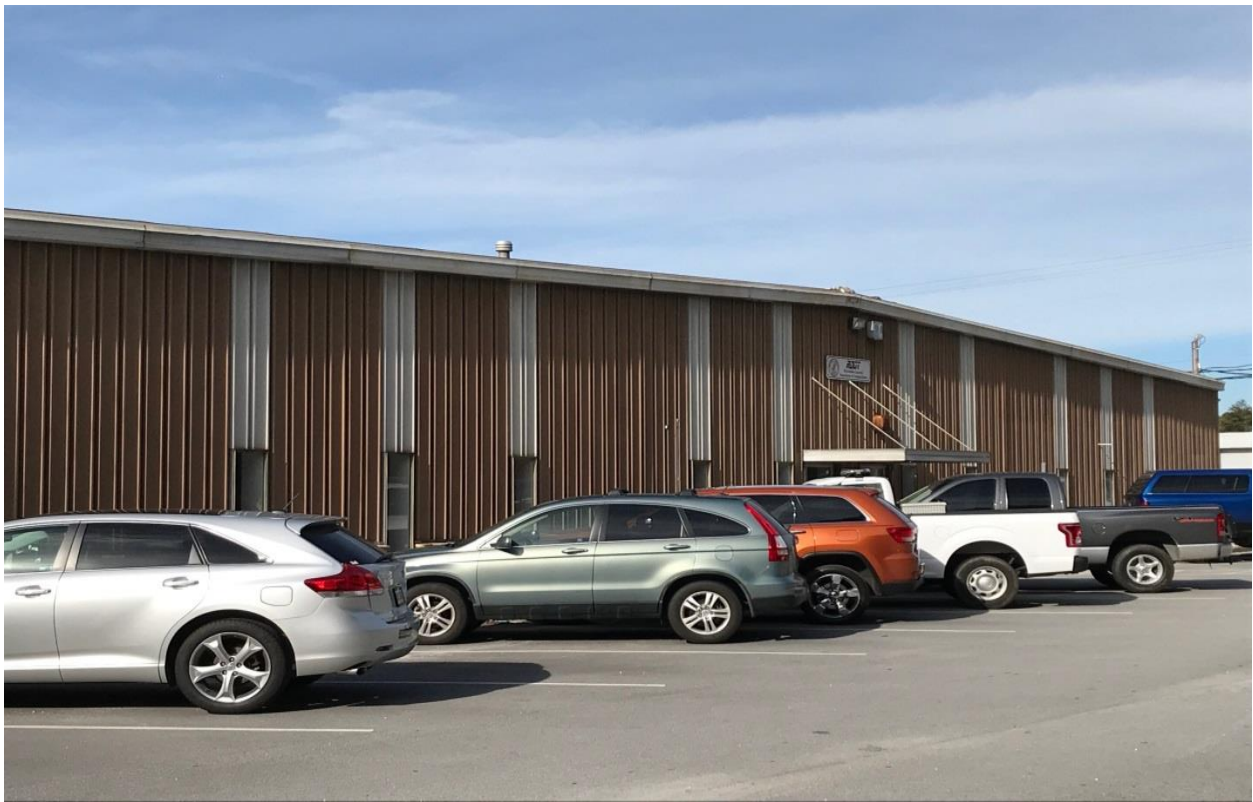
Front side of building Facing Rd.
