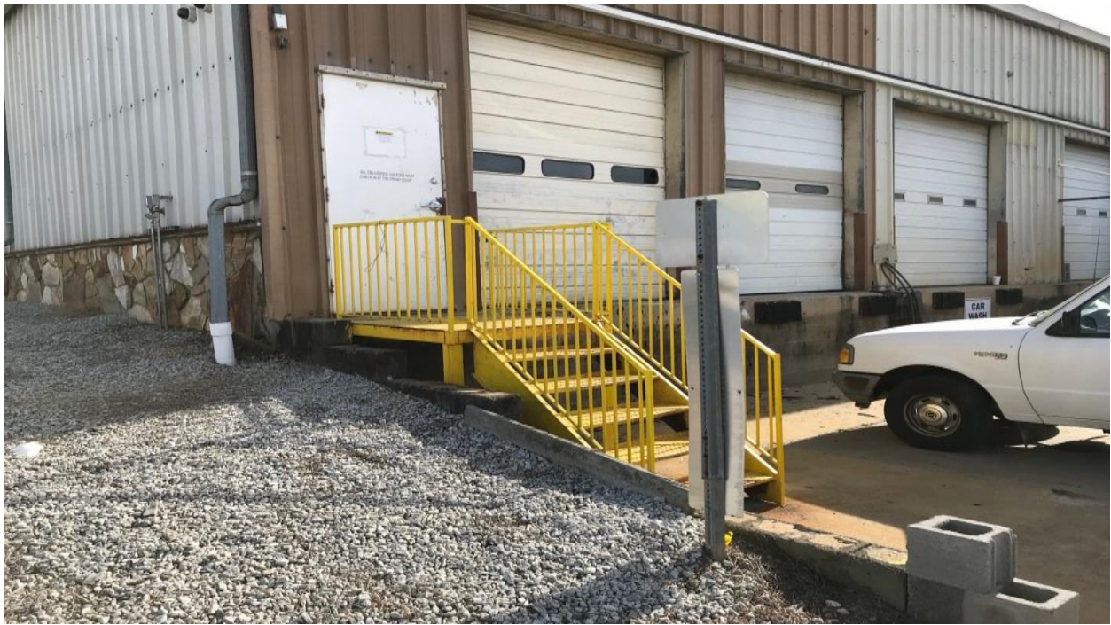
Paint Stairwells GDOT yellow
