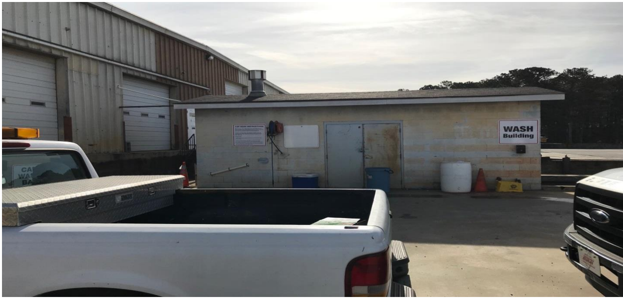
Alternates- Clean and Paint Wash Building
