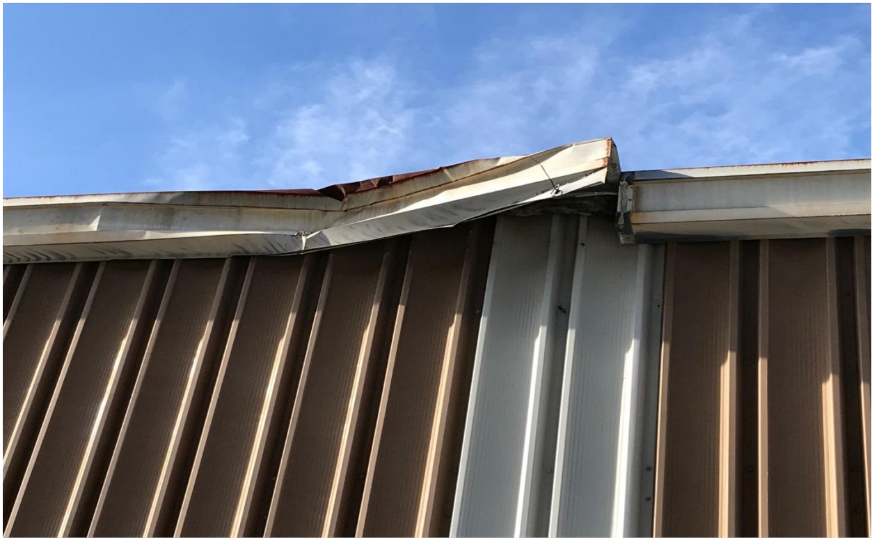
Replace Damaged Metal Framing
