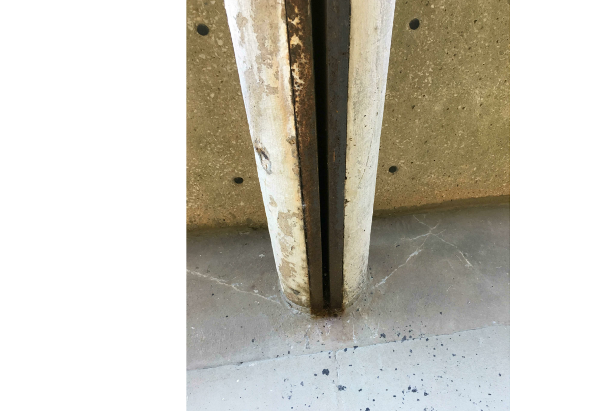
A13 Scale Column @ Exp JT Low No Scale
