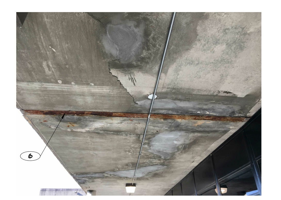
A7 Scale No Scale Bot of Elevated Walkway Exp JT
