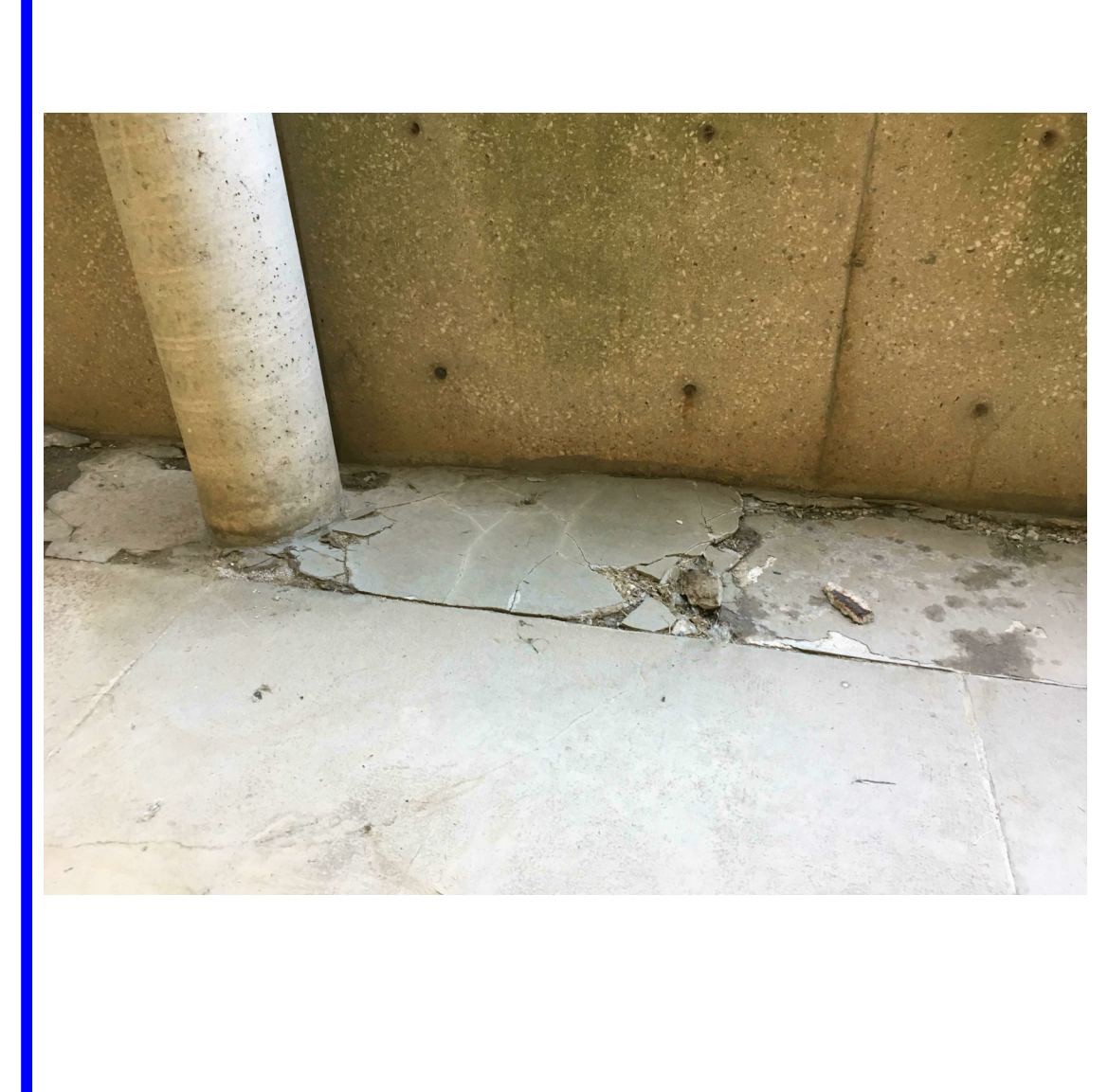
D4 Scale Slab on Grade No Scale
