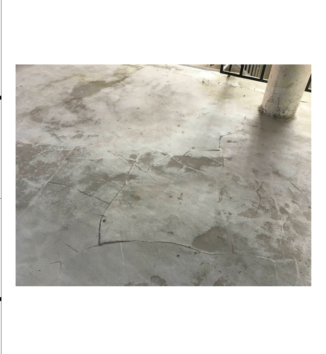
D1 Scale No Scale Top of Elevated Walkway
