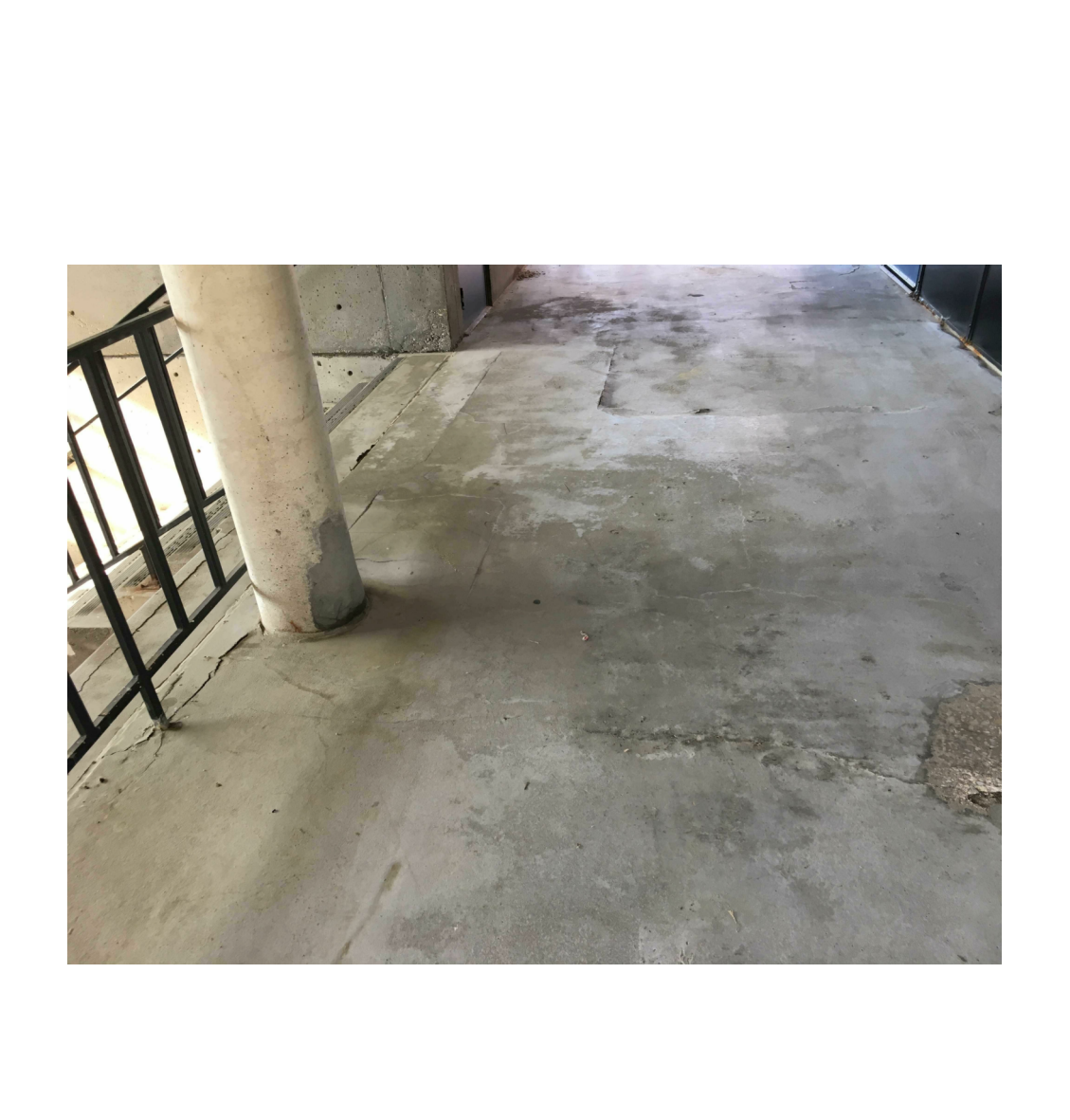
D10 Scale No Scale Top of Elevated Walkway
