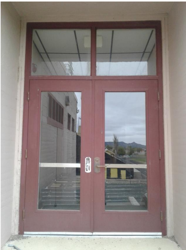
Doors 13 & 14 south exit
