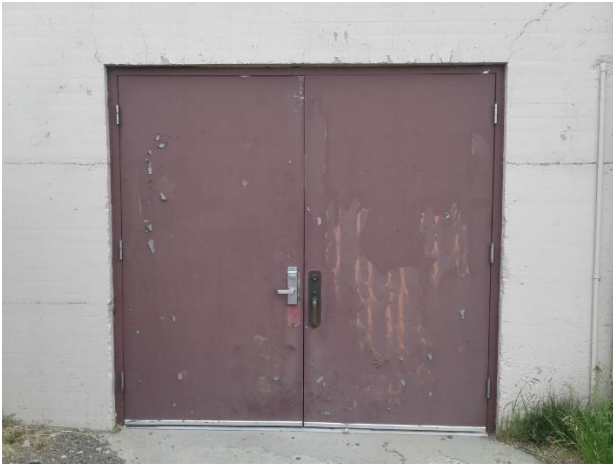
Doors 10 & 9 lower level east
