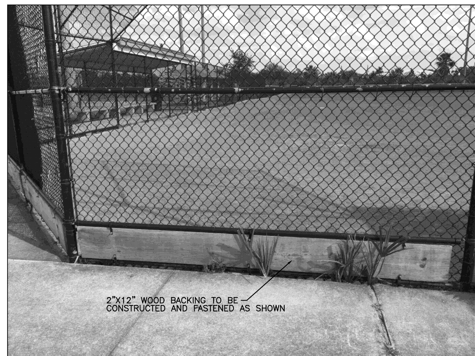
BACKSTOP WOODEN FENCE BACKING
