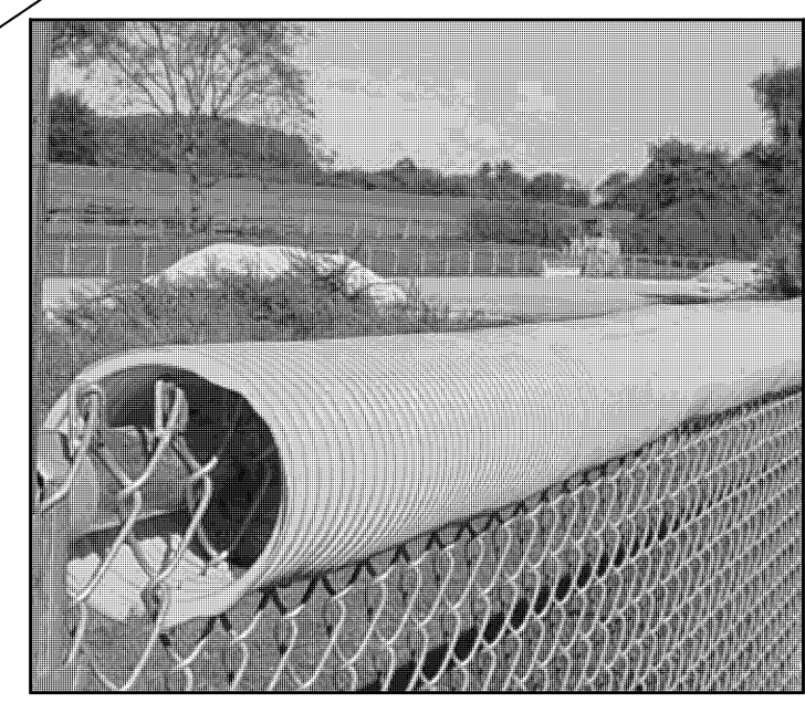
BEACON ATHLETICS ECONOMY FENCE CAP OR APPROVED EQUAL 4.5\"/> FENCE CAP DETAIL (N.T.S.)
