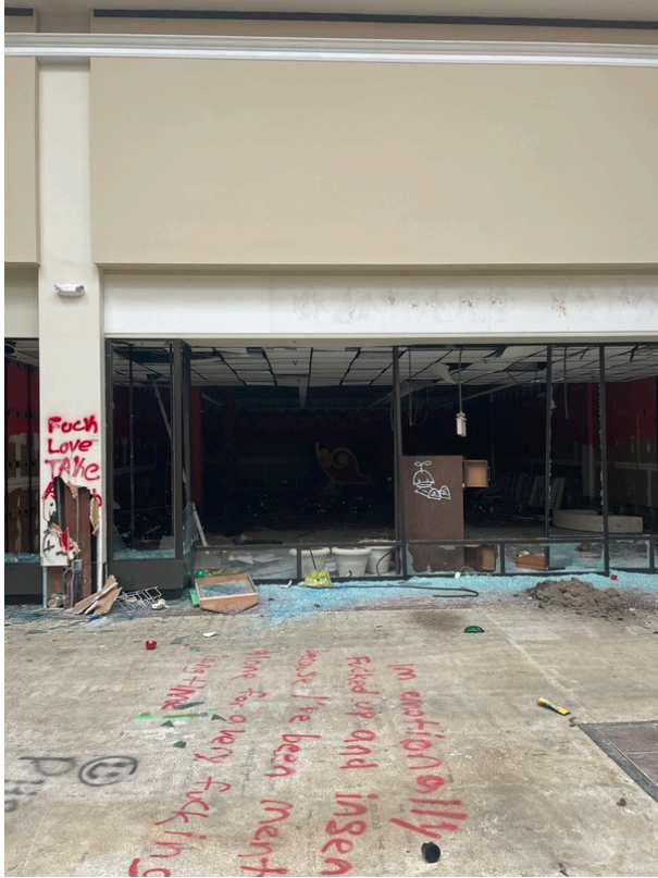
View of Room 271
