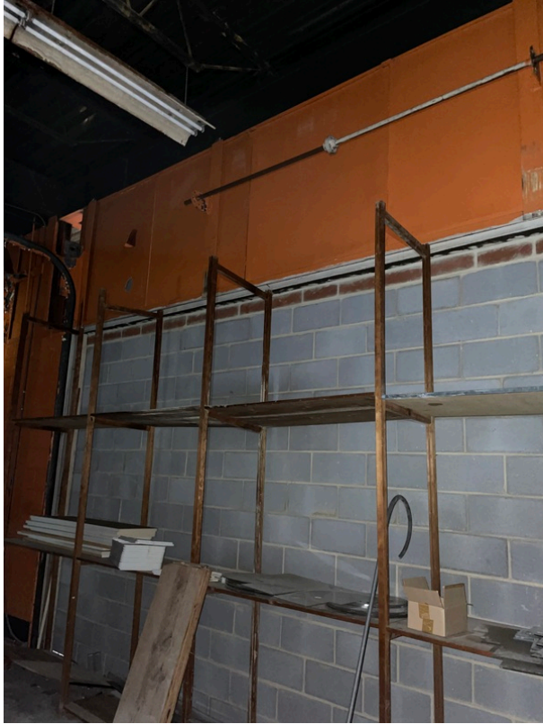
View of Transite Panels assumed to be asbestos-containing (HA 225)
