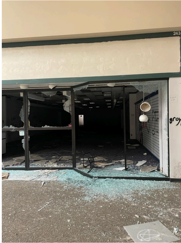
View of Room 243
