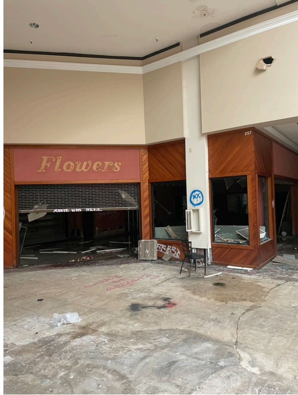
View of Room 257
