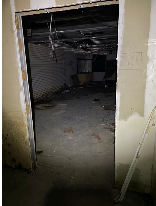
View of Room 218
