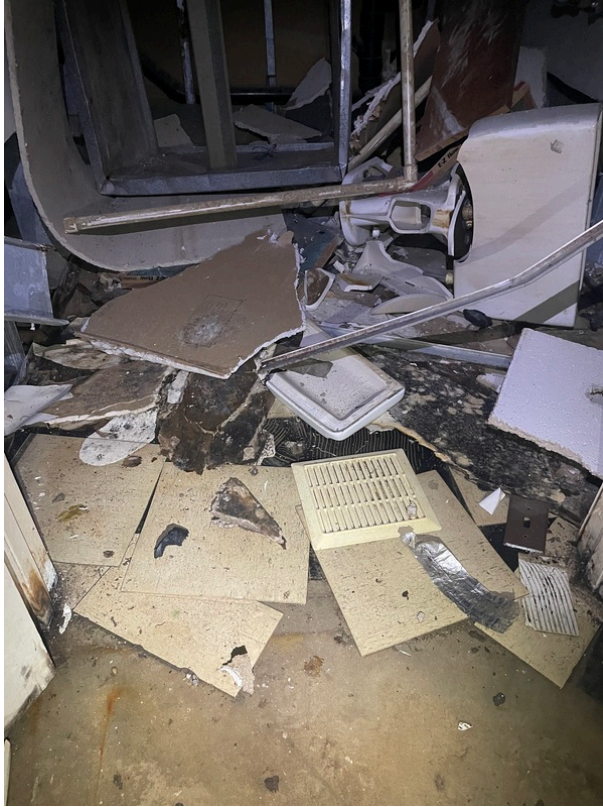
View of asbestos-containing 12" x 12" Tan Floor Tile and its associated Black Mastic (HA 165)
