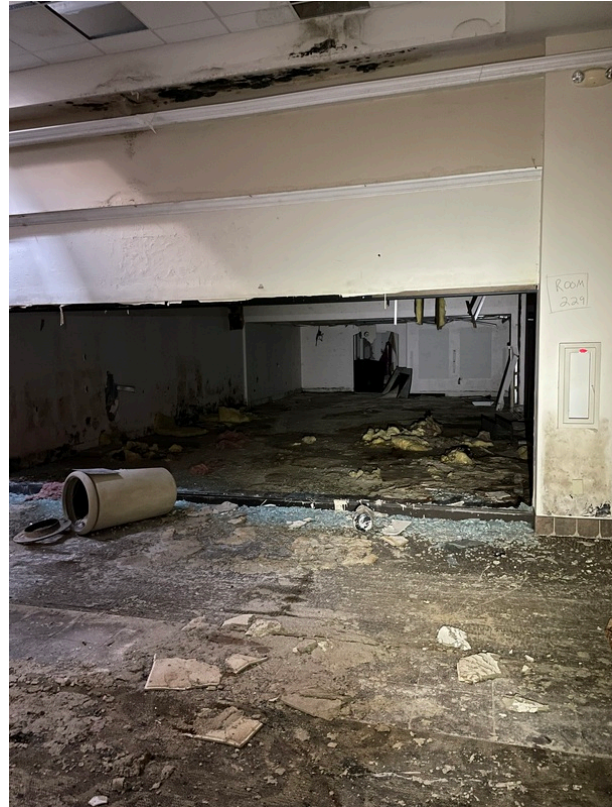
View of Room 229
