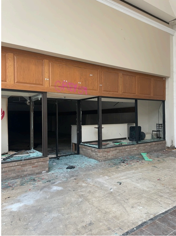
View of Room 273
