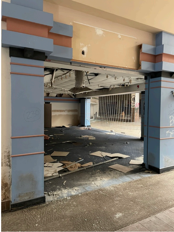
View of Room 230
