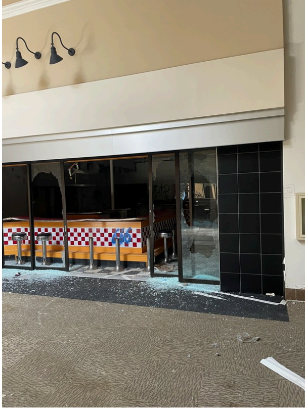
View of Room 252
