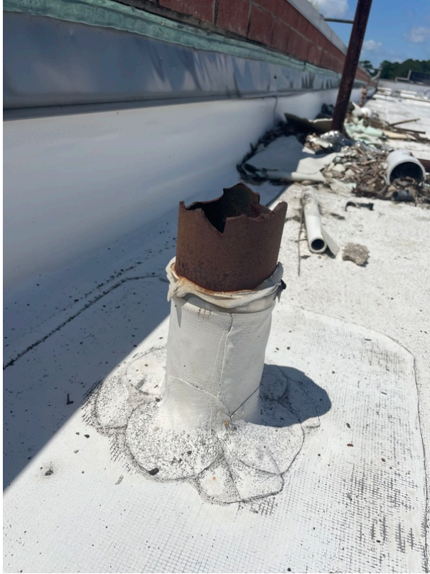
View of asbestos-containing Grey Caulk beneath Tan Caulk (HA 14)
