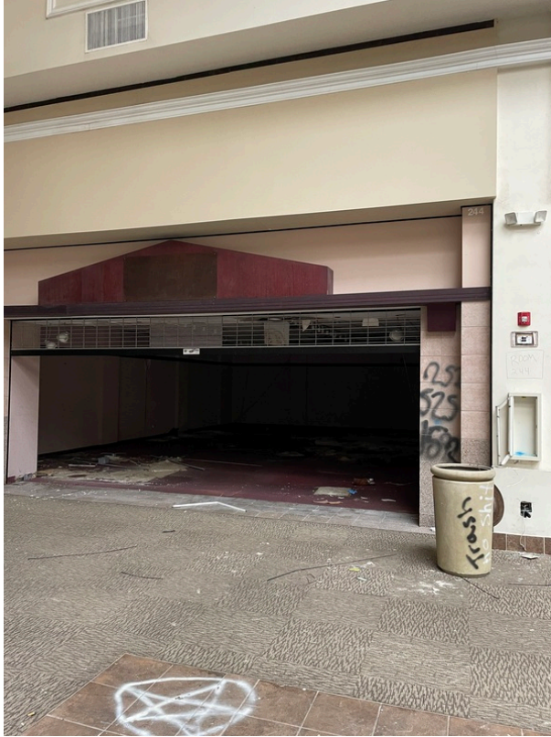
View of Room 244
