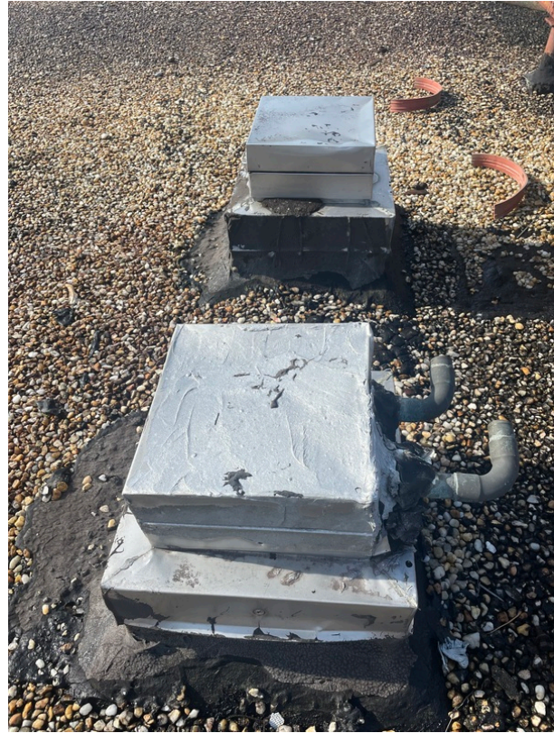
View of asbestos-containing Silver Penetration Coating (HA 4)
