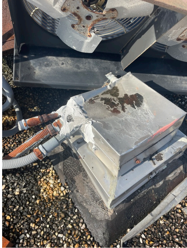
View of asbestos-containing White Penetration Caulk (HA 6)
