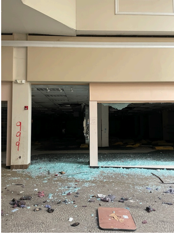
View of Room 239
