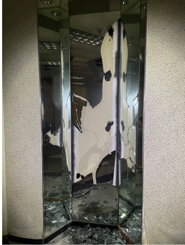
View of asbestos-containing Black Mastic Dot (HA 210)
