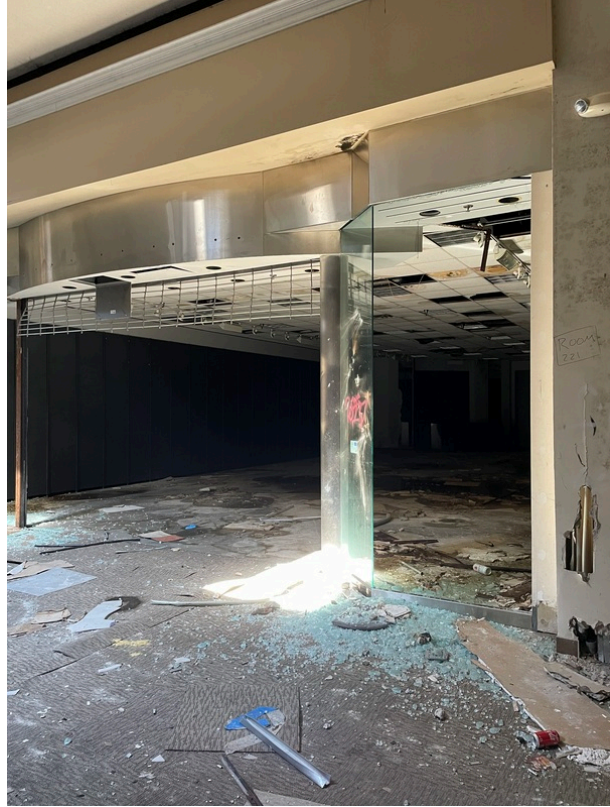
View of Room 221
