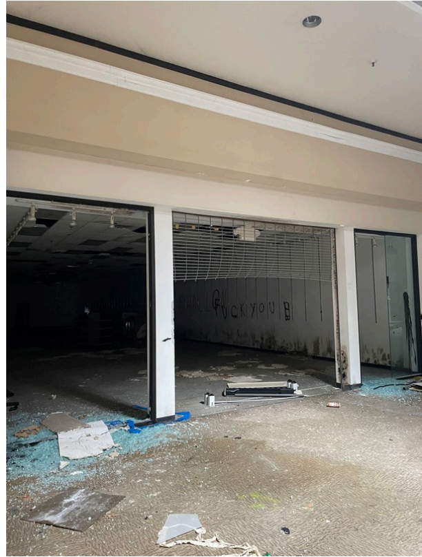
View of Room 217
