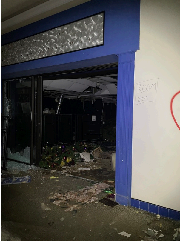
View of Room 209
