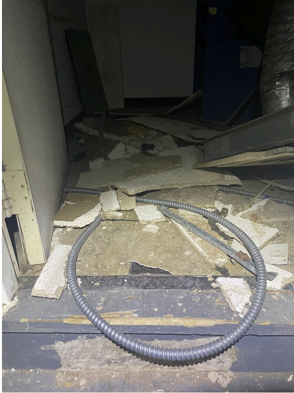
View of asbestos-containing 12" x 12" Tan Floor Tile and its associated Black Mastic (HA 153)
