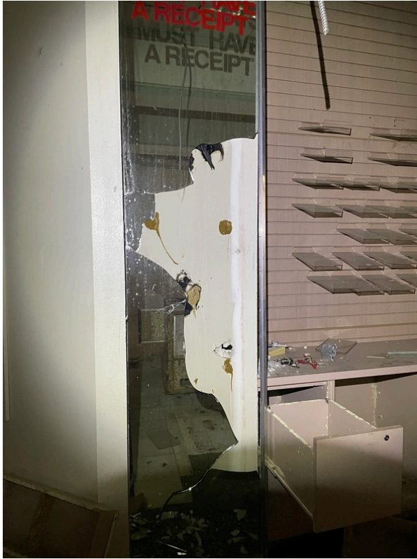
View of asbestos-containing Black Mastic Dot (HA 199)
