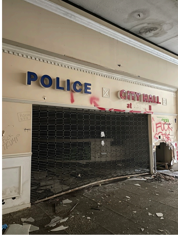
View of Room 222
