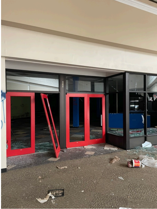
View of Room 248
