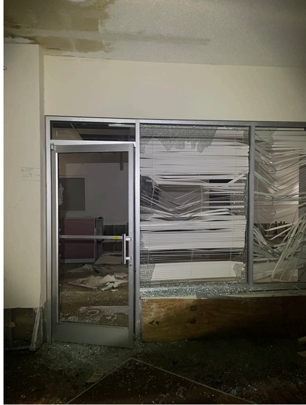
View of Room 269
