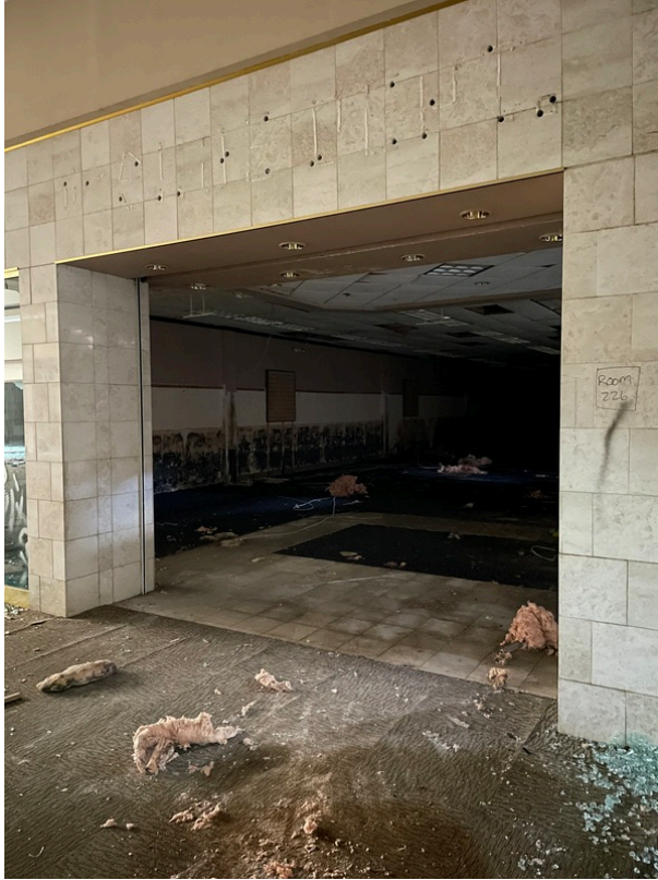
View of Room 226
