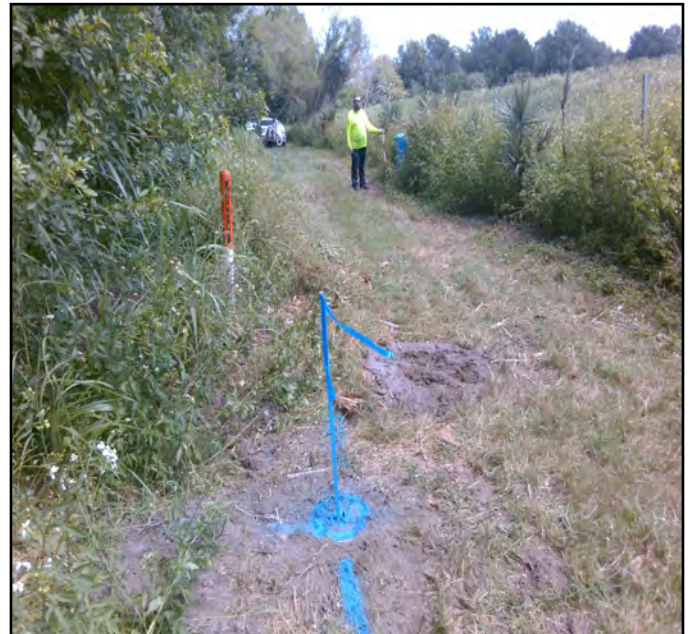
Tie 02 (From Test Hole): VALVE, WATER
