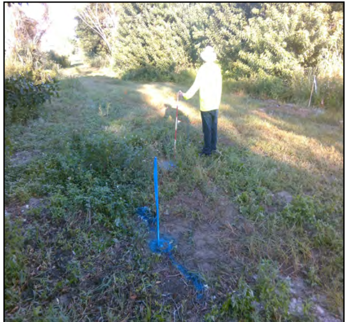
Tie 02 (From Test Hole): VALVE, WATER
