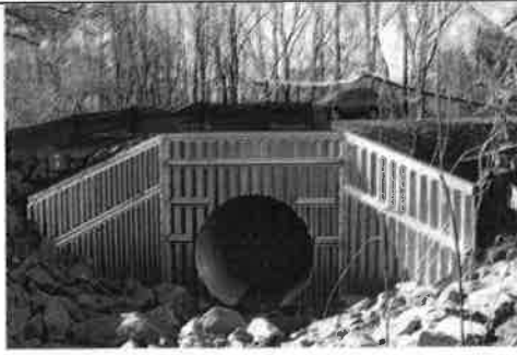
Use Pipe Wingwall
