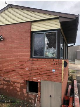
Scale house is approximate  $22' \times 18'$  with elevated first floor and basement. Masonry walls with wood truss roof and wood joist floor structures. Recommendation includes removal of structure in its entirety including utilities, back-fill of basement and repair of site, and installation of remote control for existing scale
