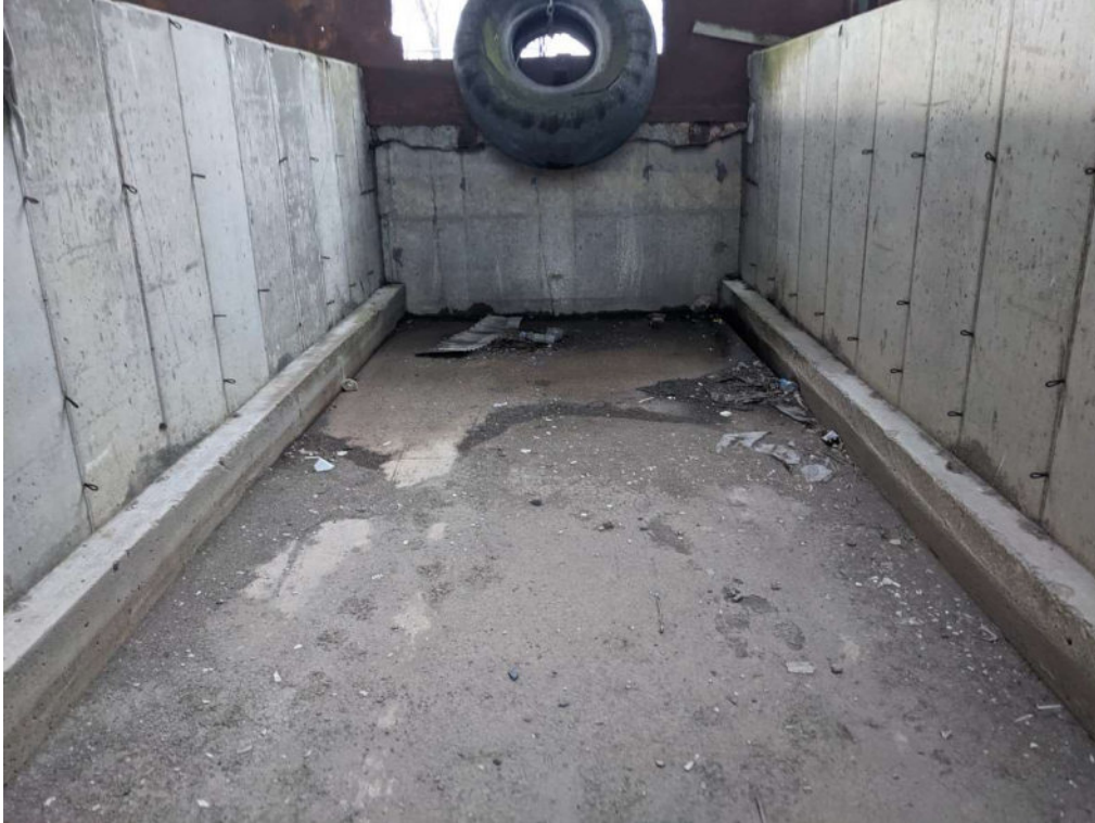
Photo 19. In Sorting Building, where trucks drive into to unload. Site A
