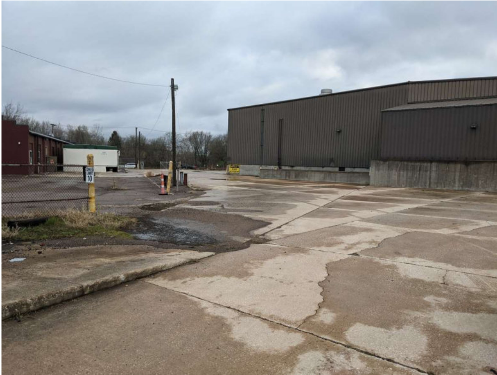
Photo 1. Facing entrance of north central side of Site A.
