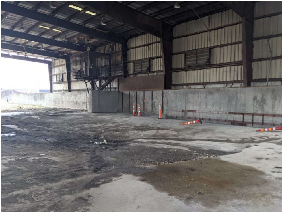
Photo 20. Transformers in cage on wall in the Sorting Building. Potential for PCBs. Staining present on floor. Site A
