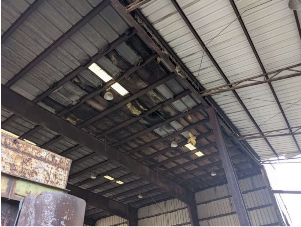
Photo 17. Ceiling in Sorting Building. Site A
