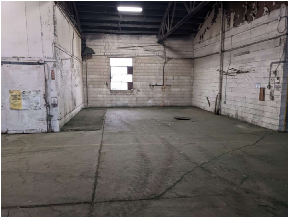
Photo 10. Oil/Water Separator in northwest section of the Maintenance Building. Outlet is unknown. Site A.
