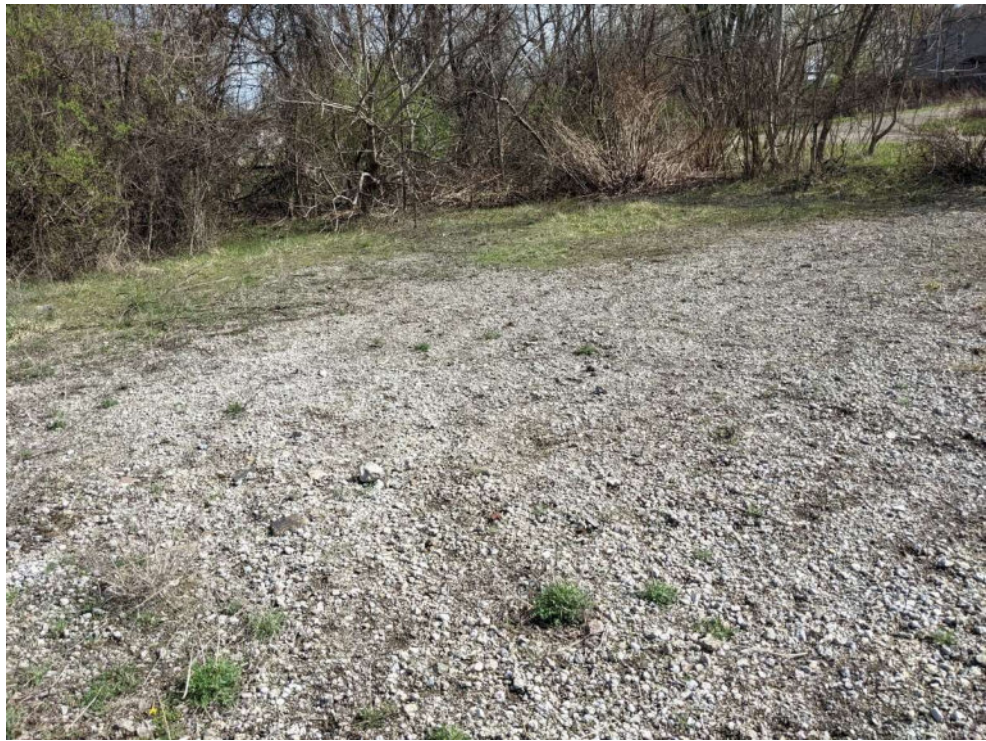
Photo 32. Gravel pad located at PN 246327. Site B.
