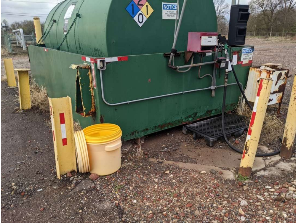
Photo 3. Close up of AST with spill kit present, some staining in area is present.
