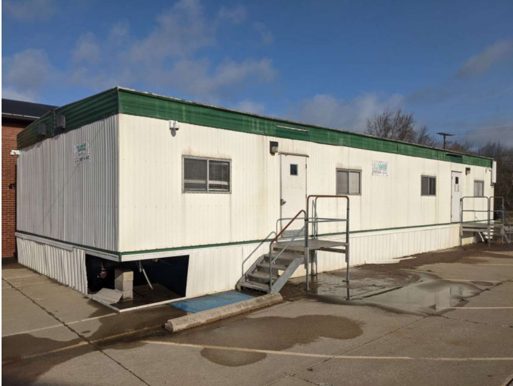
Photo 15. Pop up trailer on east side of Maintenance Building used for offices. No access was provided during assessment. Site A.
