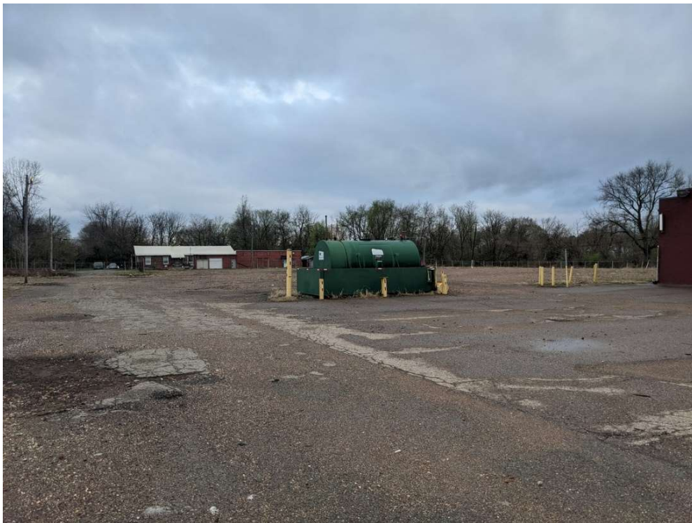
Photo 2. 6,000-gallon diesel AST located south of maintenance building-Site A.
