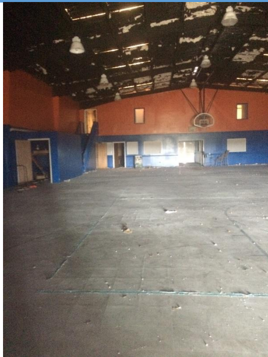
Interior view of main portion of building (basket ball court)
