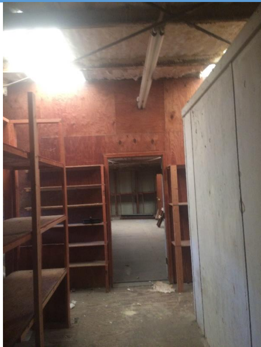
2 nd floor above offices
