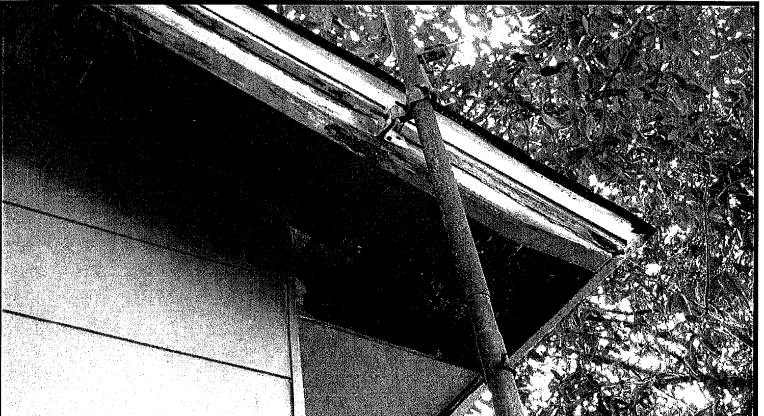
Photo No. 6: REPRESENTATIVE VIEW OF THE EXTERIOR WOOD ROOF DECK, GABLE END RAFTER AND FASCIA BOARDS THAT ARE COATED WITH LEAD-BASED PAINT.
