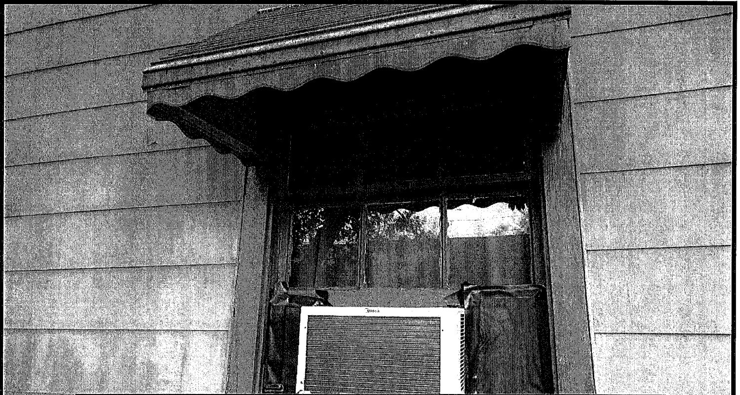
Photo No. 5: REPRESENTATIVE VIEW OF THE EXTERIOR WOOD WINDOW ASSEMBLIES THAT ARE COATED WITH LEAD-BASED PAINT.
