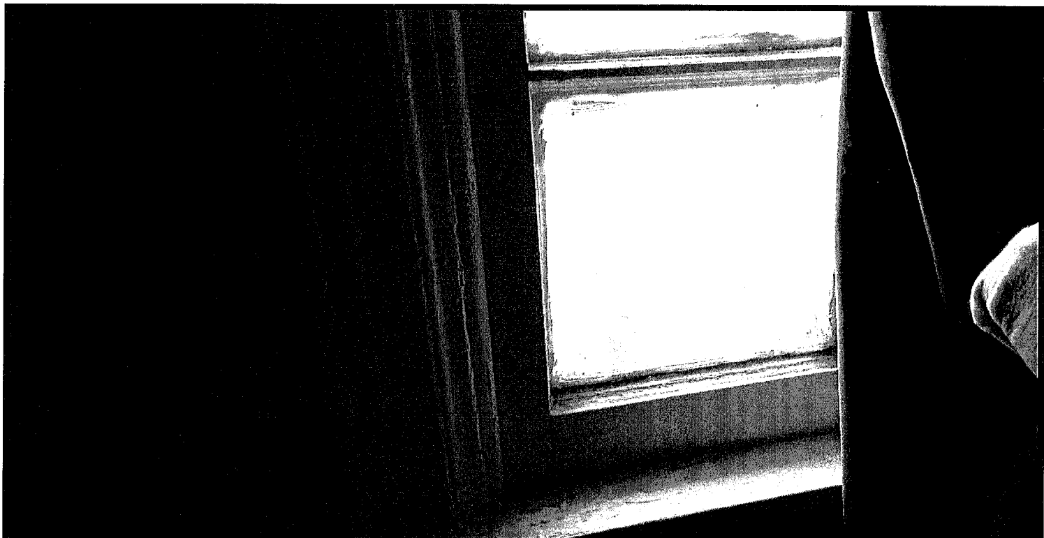
Photo No. 3: VIEW OF THE WHITE WOOD WINDOW ASSEMBLY IN THE BATHROOM THAT IS COATED WITH LEAD-BASED PAINT. THE DOOR CASING IS ALSO COATED WITH LEAD-BASED PAINT.
